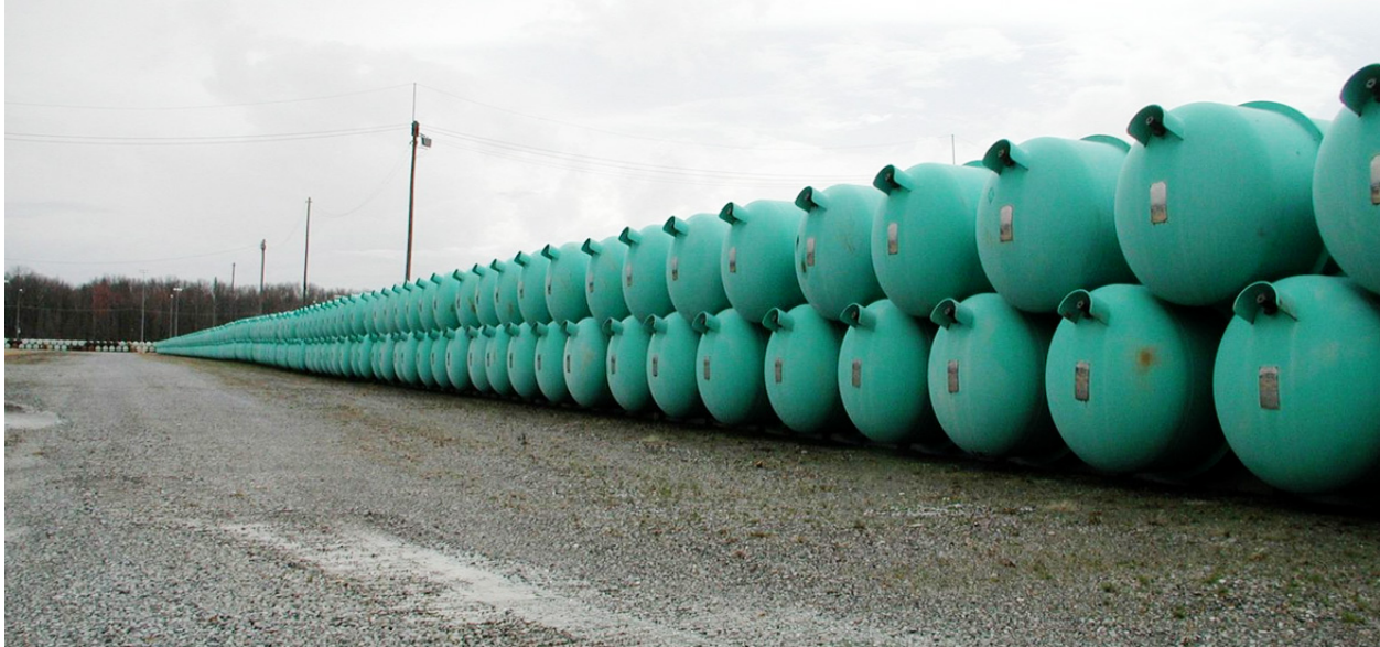
Figure S-4 Depleted Uranium Hexafluoride Cylinder Storage Yard (Source: BWXT 2016)
