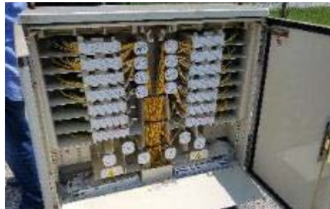
Photographs of optical fiber patch panel at EPB's Riverside and Tennessee Tech power distribution substations. Duplex SMF28e+ single mode fiber with LC terminators.
