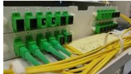
Photographs of optical fiber patch panel at EPB's Riverside and Tennessee Tech power distribution substations. Duplex SMF28e+ single mode fiber with LC terminators.
