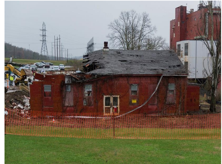
Y-12 Biological Facility Progress
