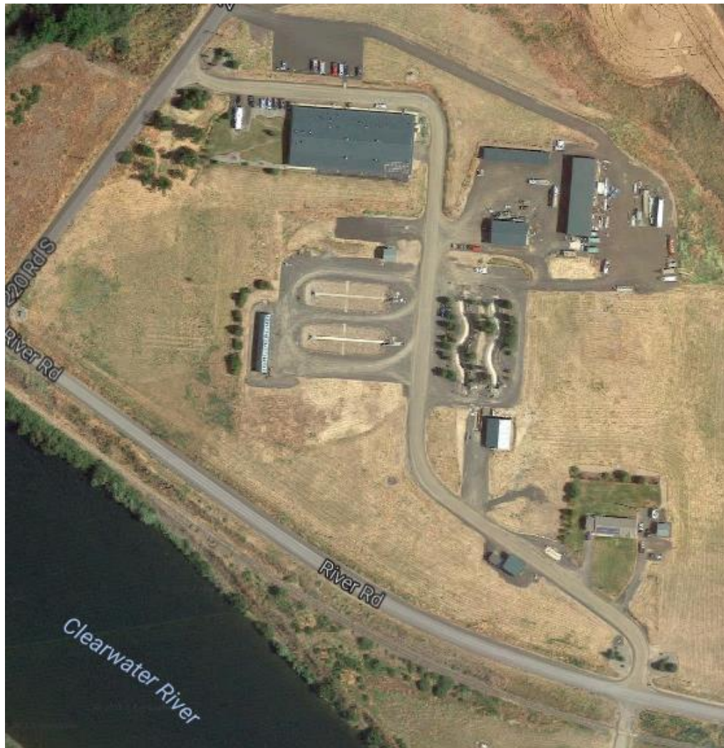
Figure 5 Existing facilities at NPTH
