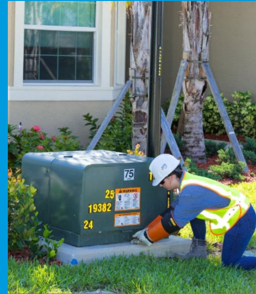
Storm Secure Underground Program
