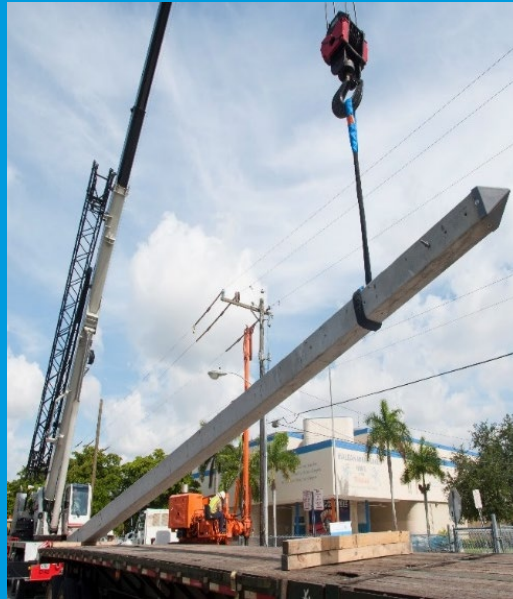
Building on proven hardening investments
