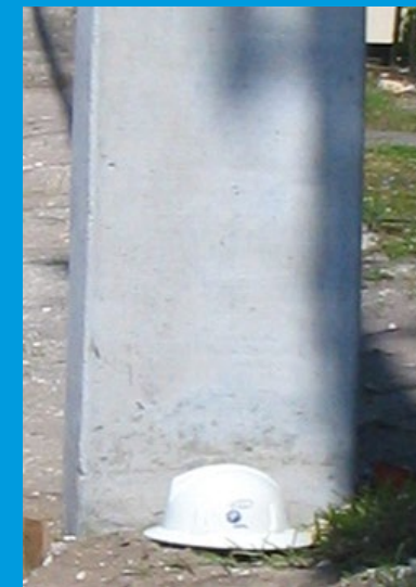
55' IIIH Cast Concrete
