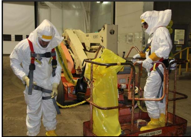
ITG employees ensure fall protection equipment is securely in place, left, before starting operations to change air filters on the Retrieval Containment Enclosure, below, which is located inside the Transuranic Storage Area-Retrieval Enclosure that houses the remaining stored legacy radioactive waste
