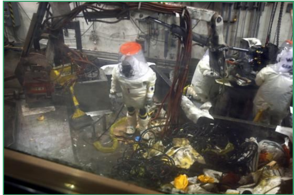
Remediation of south boxline required numerous cell entries by employees in Type "B" bubble suits.
