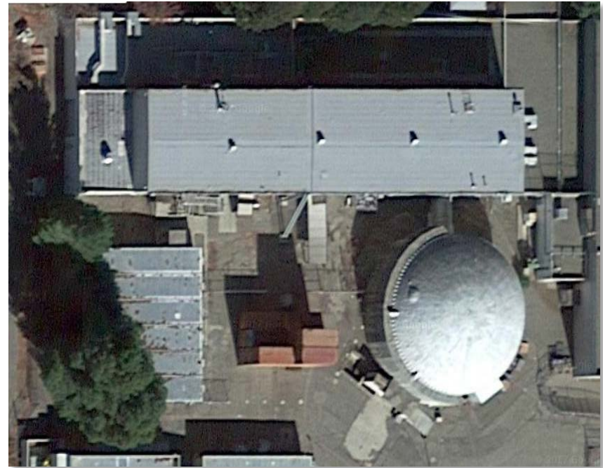
LLNL– Livermore Pool Type Reactor Building 280
