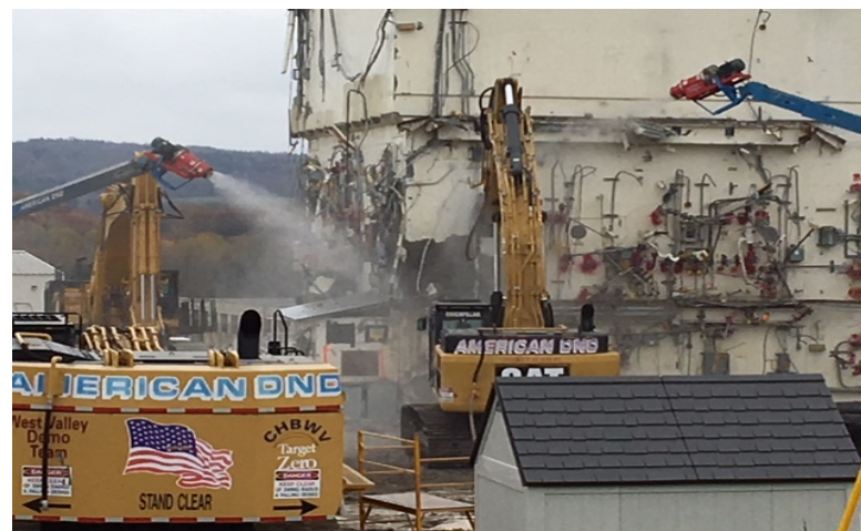
Demolition of WVDP Vitrification Facility
