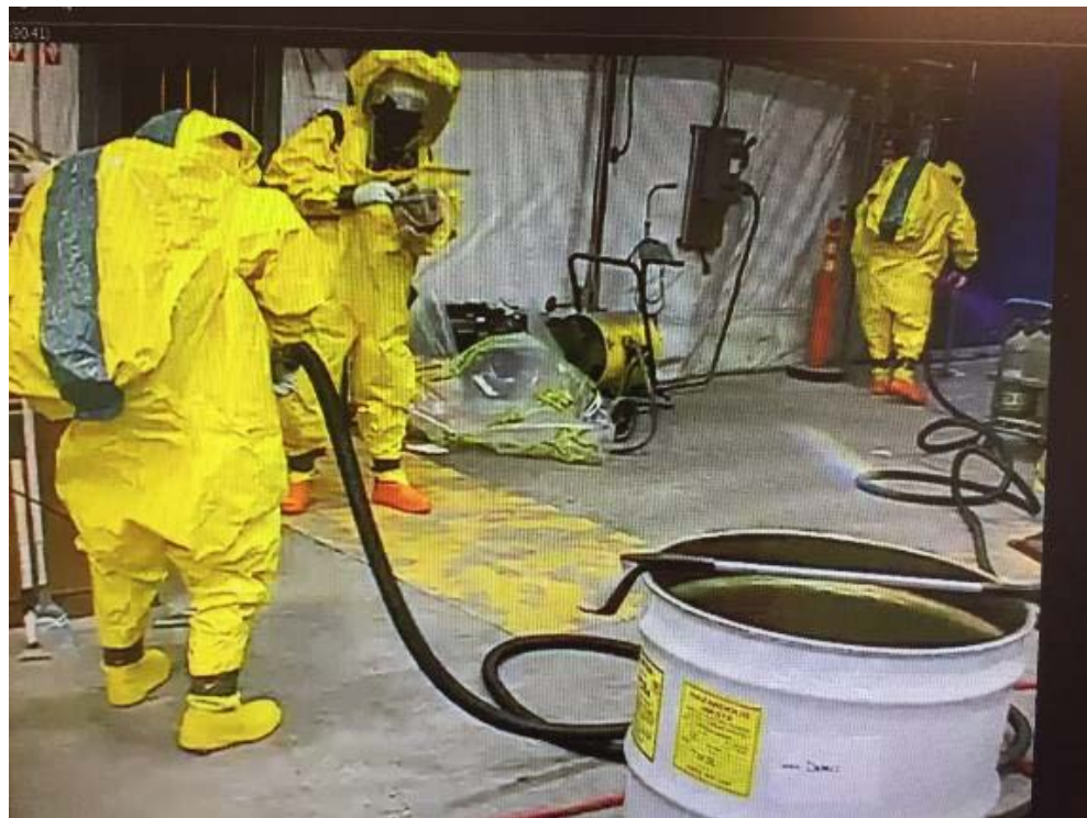
(Above) workers in Anti-contamination clothing clean up loose material from the ARP V airlock floor
