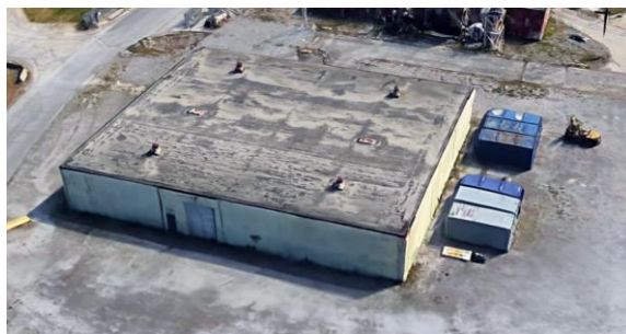
Y-12 National Security Complex – Beta-4 Tool Storage Facility
