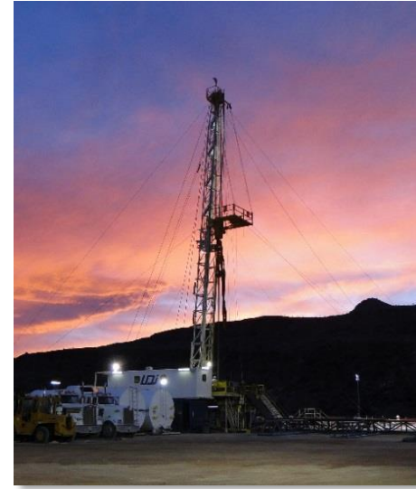
Groundwater Well Drilling
