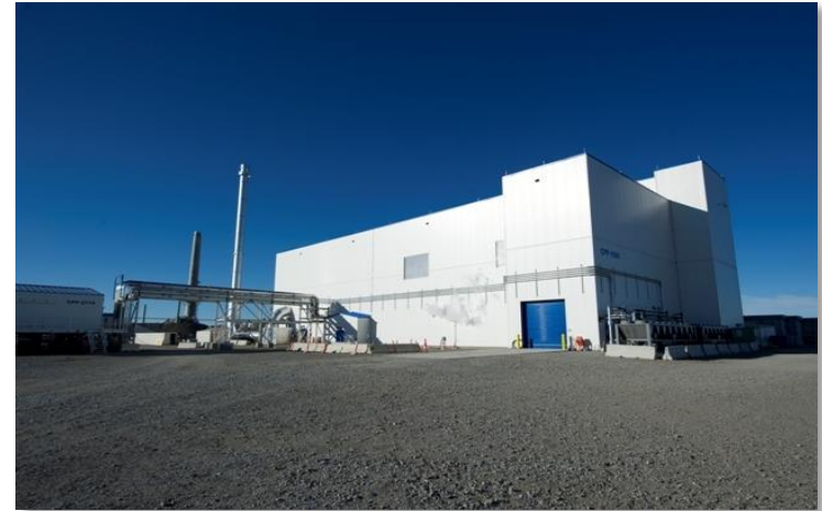
Integrated Waste Treatment Unit
