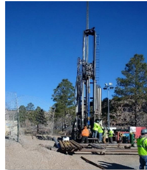
Chromium project extraction wells at Los Alamos, New Mexico
