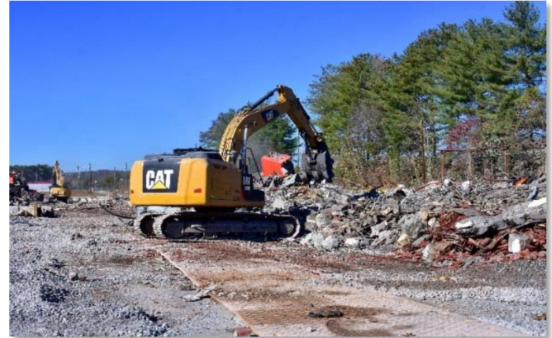
Demolition of East Tennessee Technology Park facilities
