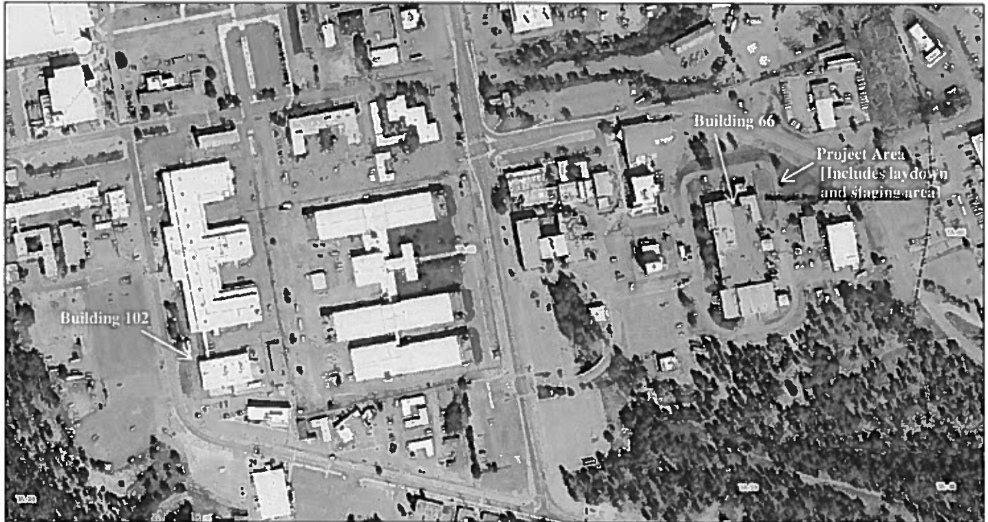
Figure 1: Buildings 102 and 66 at TA-3
