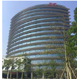
Singyes Solar HQ building
