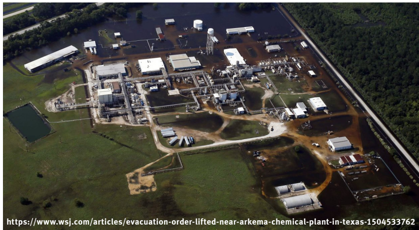
Figure 2. The flooded plant of French chemical maker Arkema SA, which produces organic peroxides, after fires were reported at the facility in Crosby, Texas, on August 31, 2017
