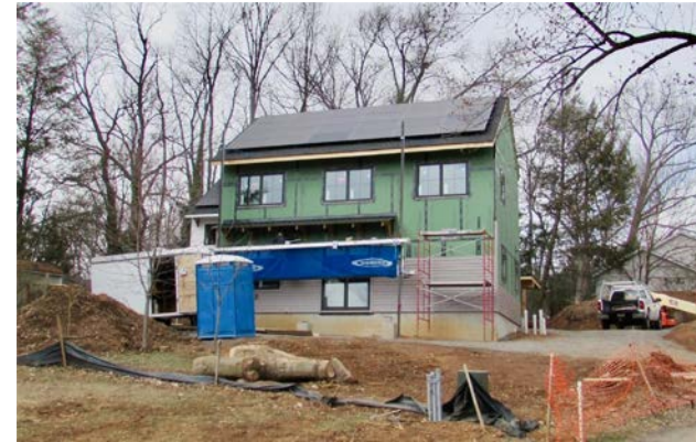
2018 GreenBuild Duplex Under Construction
