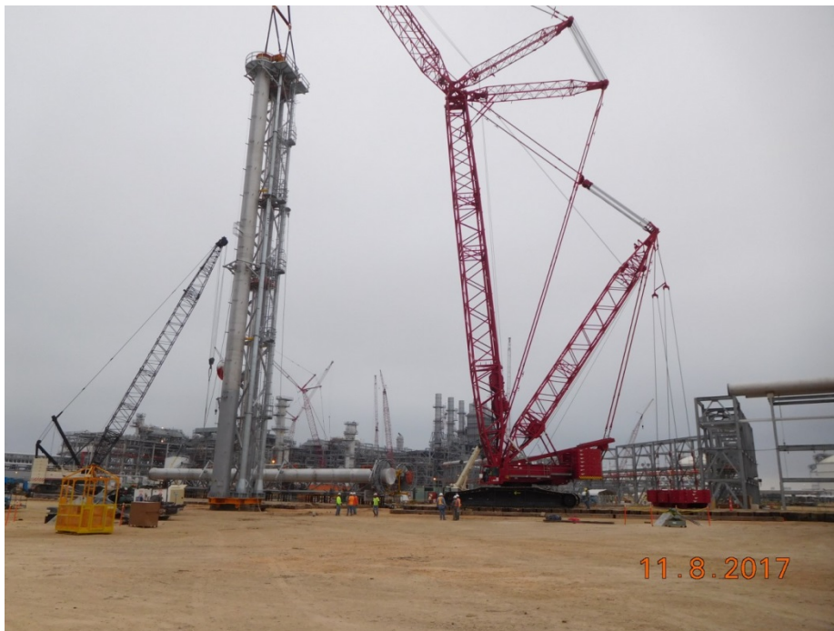
OSBL – Stage 3 Flare Bottom Section Setting
