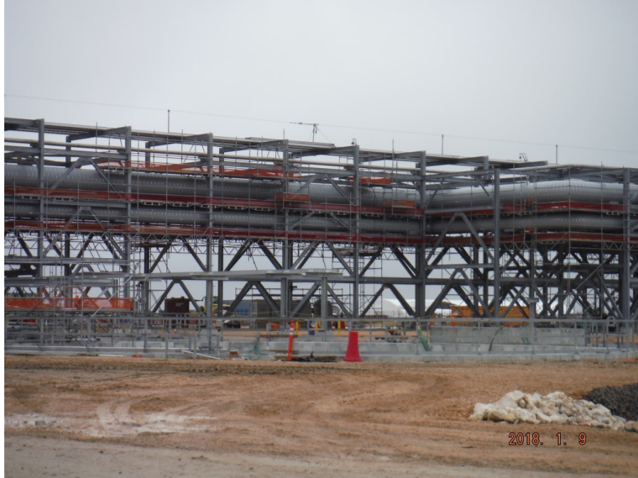
OSBL – Piping Insulation Progress
