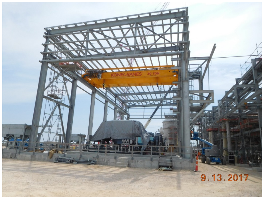
Stage 3 OSBL – BOG Compressor Building
