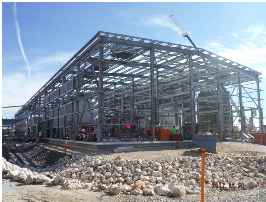
ISBL – Water Treatment Area Progress
