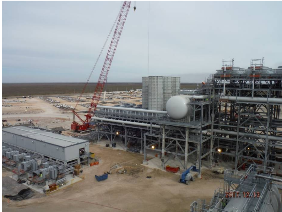
Train 5 – Installation of Propane Refrigeration Subcooler Shroud
