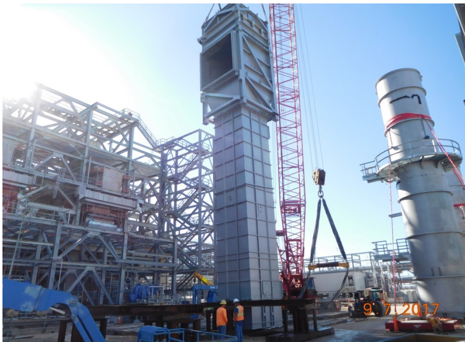
Train 5 - Gas Turbine Stacks Installation in Compressor Area
