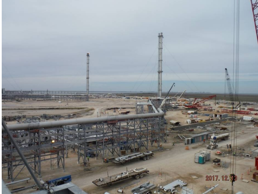
OSBL – Pipe Installation towards flare in progress
