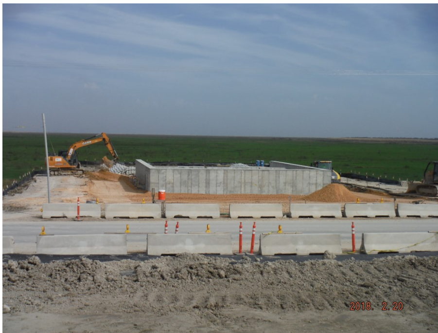
OSBL – Outfall Outlet Structure Progress
