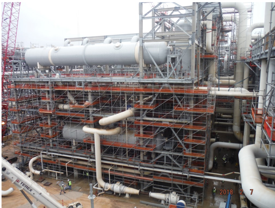
Train 5 – Piping Progress at Propane Refrigeration Area
