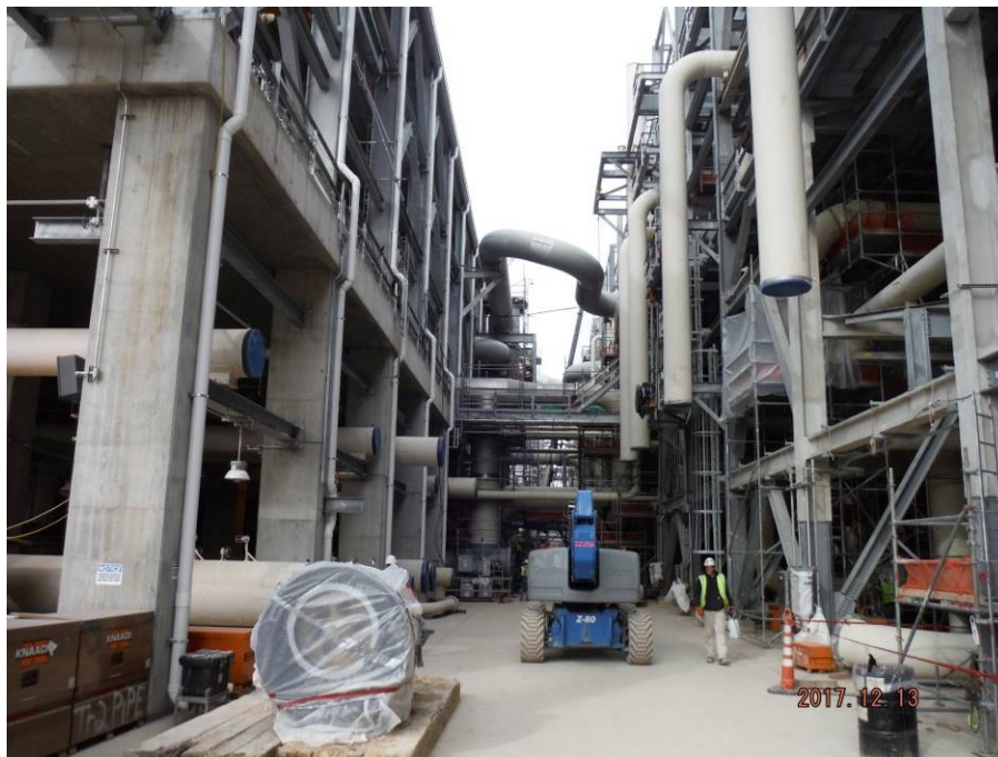
Train 5 – Piping Progress between Refrigeration Compressor Area and Cryo Pipe Rack
