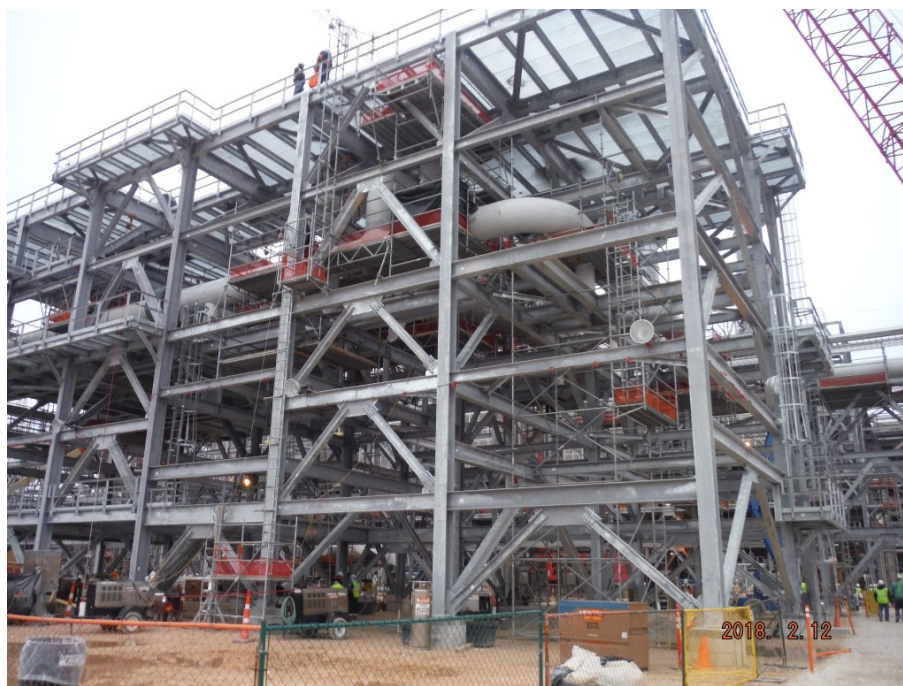
OSBL – Valve Platform Structure with Pipe Installation
