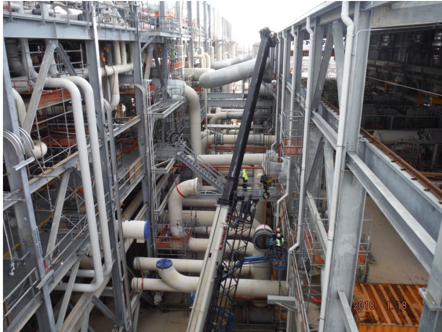
Train 5 – Piping Installation Progress at Compressor Alleyway
