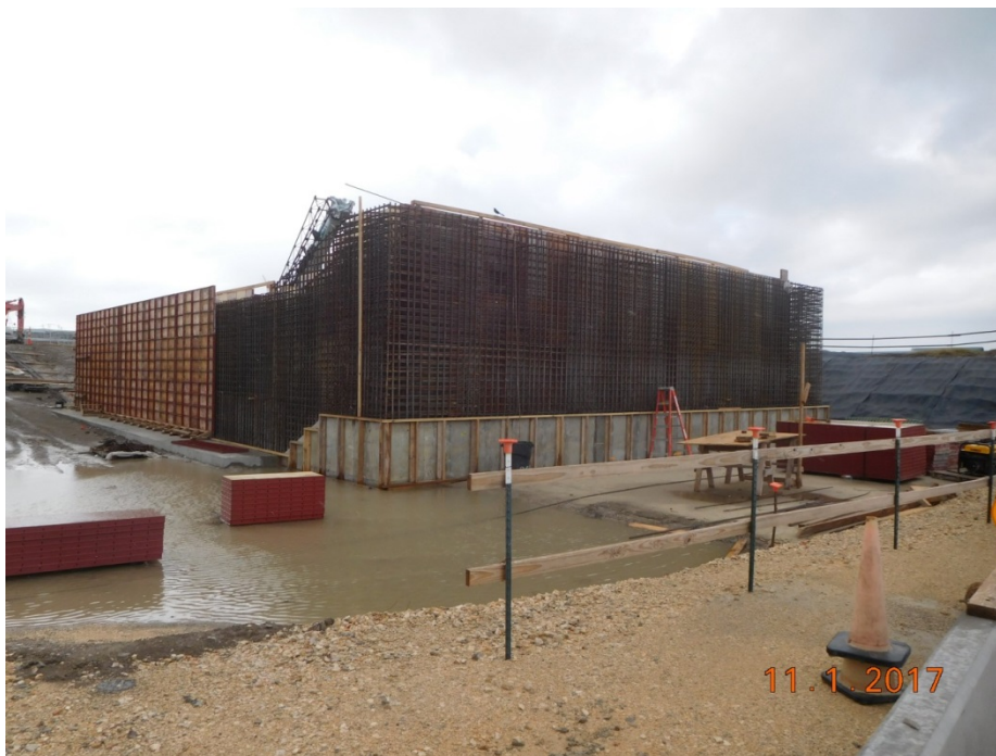
OSBL – Outfall Structure
