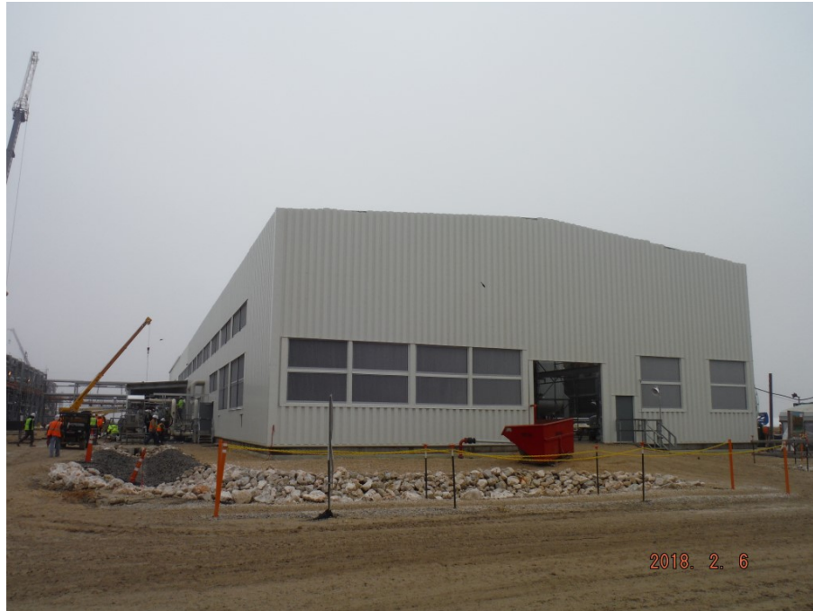
OSBL – Water Treatment Building Progress
