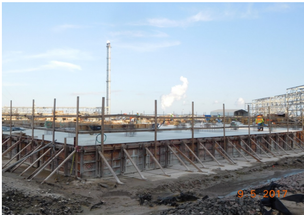
Stage 3 OSBL – Compressors Foundation - Flare Modification Scope
