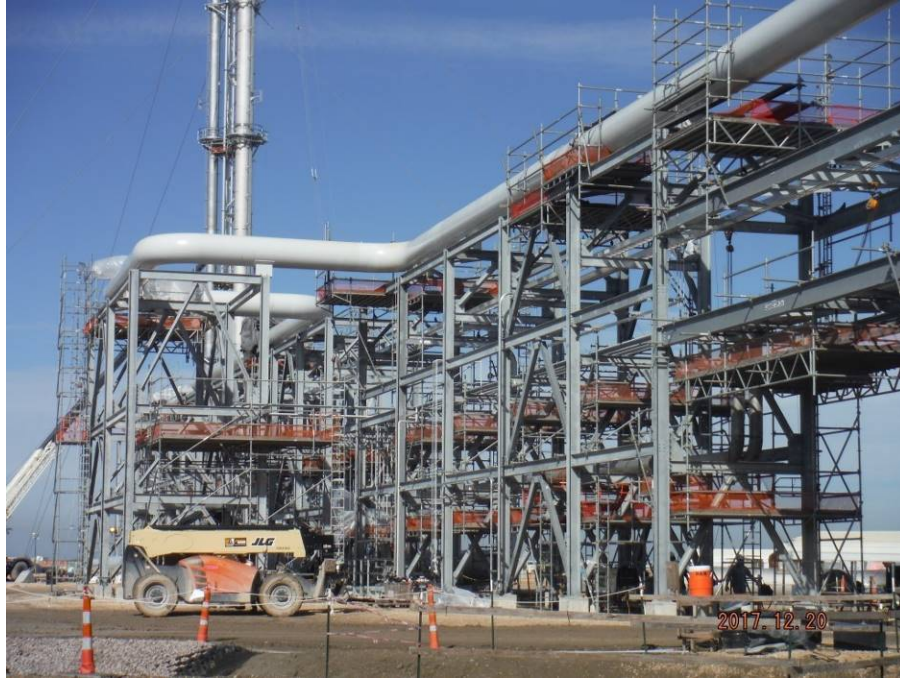
OSBL – Piping Installation towards the Flare
