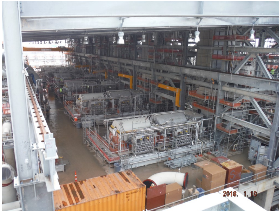
Train 5 – Construction Progress on Compressor Deck
