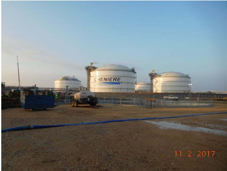
OSBL – Containment Basin
