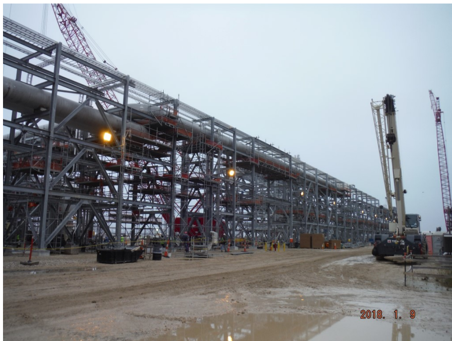
OSBL – Cable Tray Installation at R06 Pipe Rack
