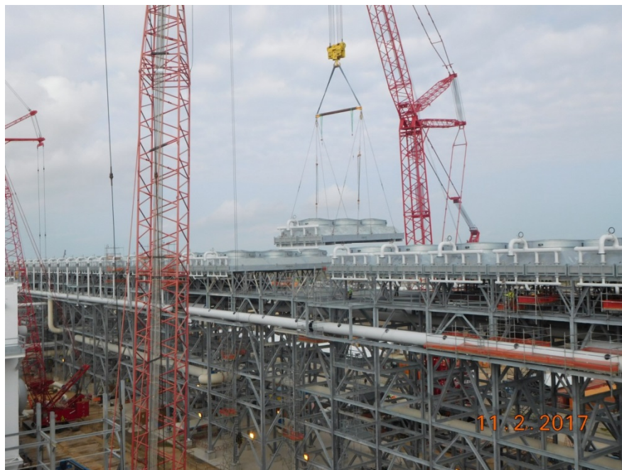
ISBL – Setting of Last Refrigeration Fin Fan
