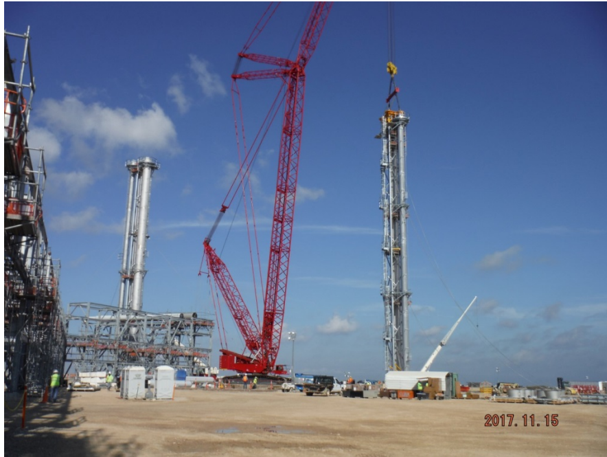
OSBL – Stage 3 Flare Top Section Setting
