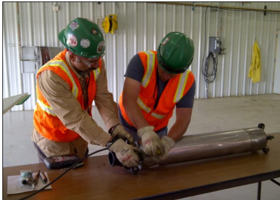
Spare leachate pump performance check installation of new level sensor
