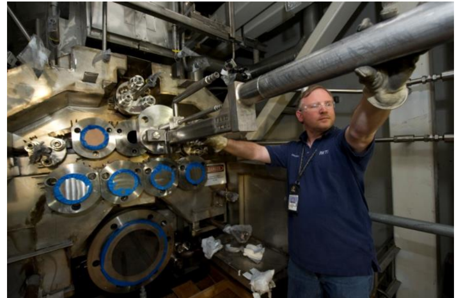
Installing the DMR waste feed spray nozzles
