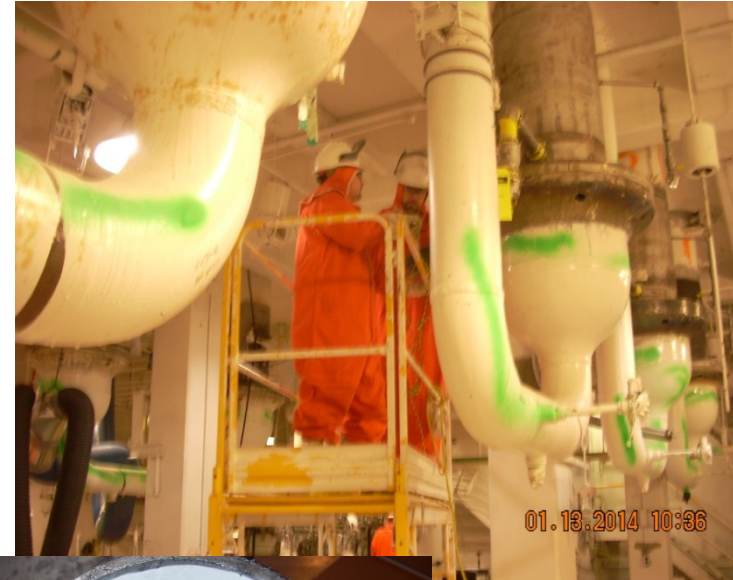
Removal of sodium-contaminated piping
