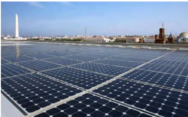
Solar panels on the roof of DOE's Forrestal Building in Washington, DC. Photo: DOE
