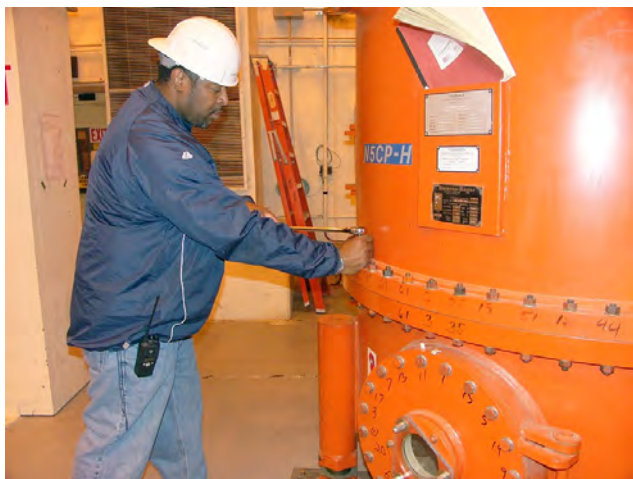
At DOE's Princeton Plasma Physics Laboratory, a technician tightens seals on a high-voltage enclosure to prevent sulfur hexafluoride leaks.
