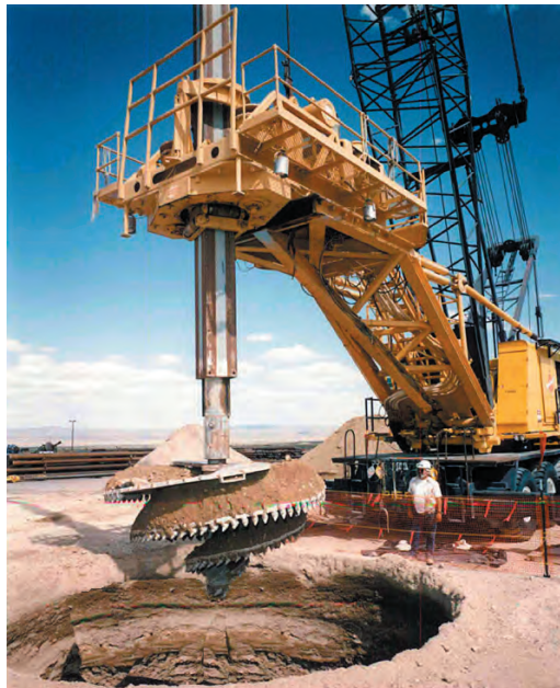
Intermediate depth boreholes are typically drilled to more than 98 feet.
