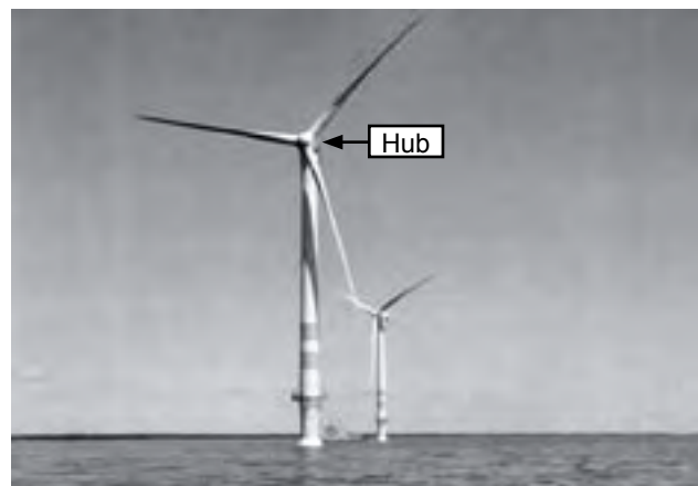
Computer-generated image of typical offshore wind turbines.
