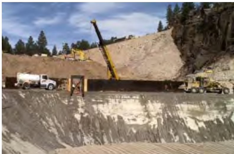
A 70-foot-high retention structure, shown here under construction by the U.S. Army Corps of Engineers, is among the DOE actions taken in response to the Cerro Grande Fire at Los Alamos.
