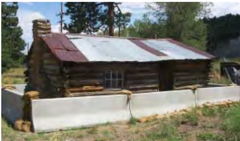
Newly installed concrete barriers protect the historic Pond Cabin from potential stormwater damage. The cabin, built in 1914, is listed on the New Mexico State Register of Historic Places.
