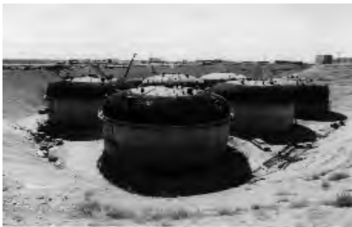
As a result of analyses conducted during the NEPA process, DOE decided not to construct six new high-level waste tanks similar to these shown under construction at Hanford during the 1970's, saving over $400 million.
