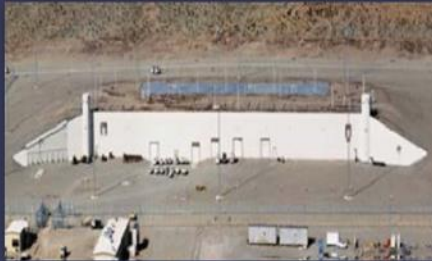
Device Assembly Facility (DAF)
