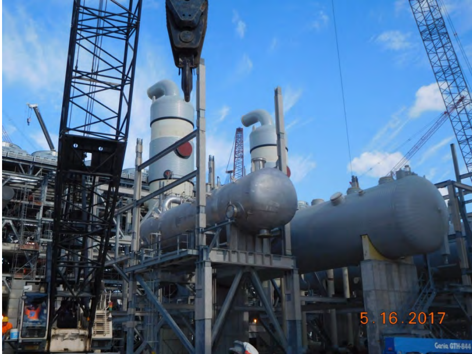
Train 5 – Ethylene Surge Drum Set in Propane Refrigeration Area
