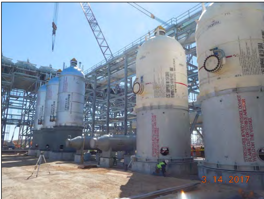
Train 5 – Mercury Removal Area Vessels Setting
