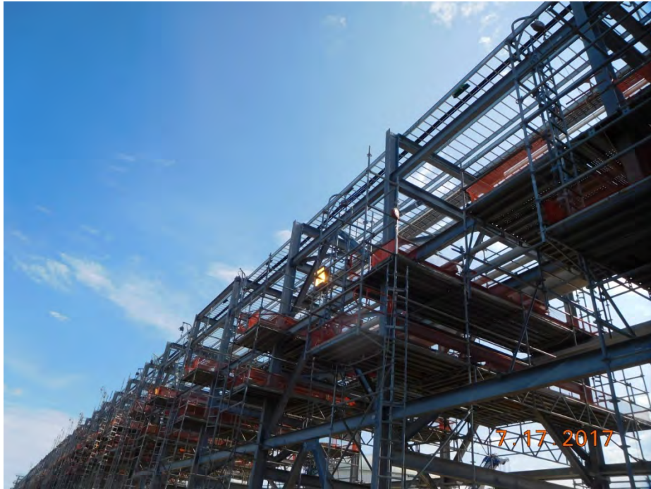
Stage 3 OSBL – 13.8 kV High Voltage Cable Pulls
