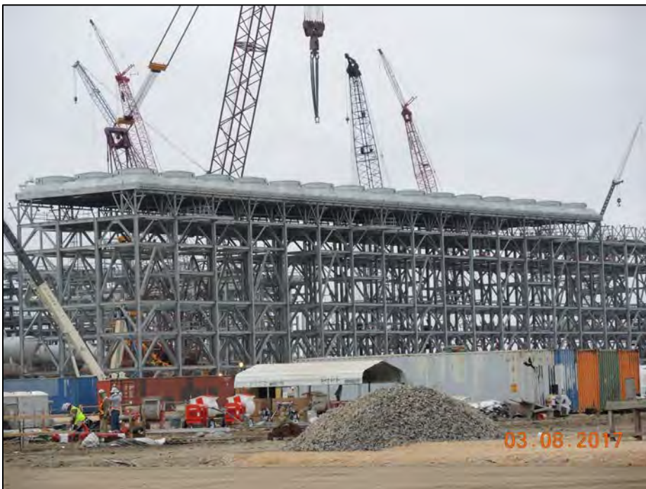
Train 5 – Propane Condenser Rack Air-Cooled Exchangers Installation
