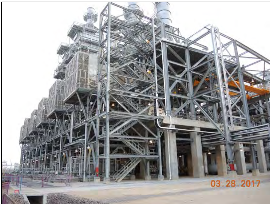
Train 3 – Compressor Area
