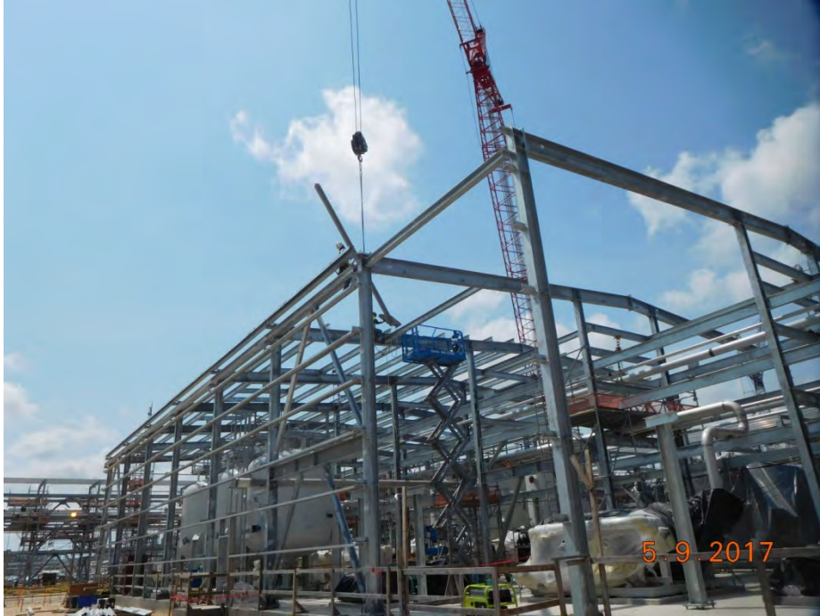
Stage 3 OSBL – Steel Erection for Water Treatment Building
