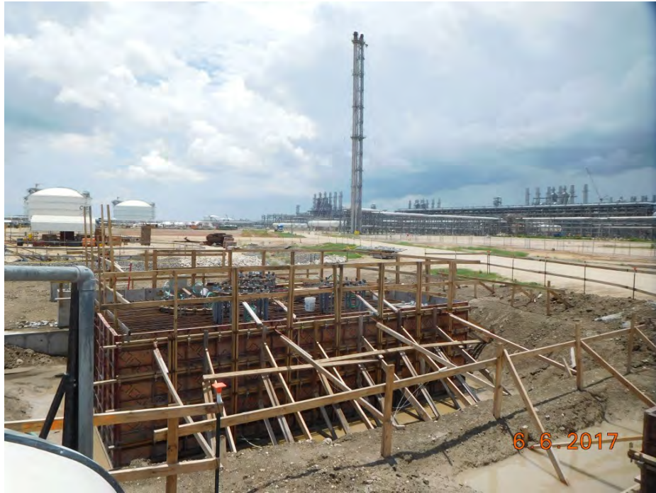
Stage 3 OSBL – Flare Base Foundation Ready to Pour Concrete
