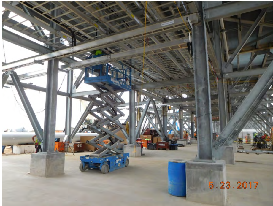
Train 5 – Installing Cable Tray in Propane Condenser Rack
