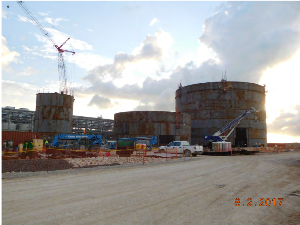
Stage 3 OSBL – Water Storage Field Erected Tanks
