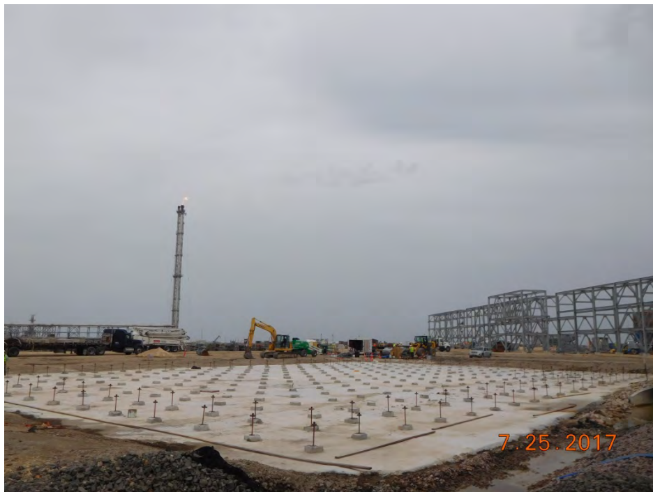
Stage 3 OSBL – Flare Modification Scope - Compressors Foundation
