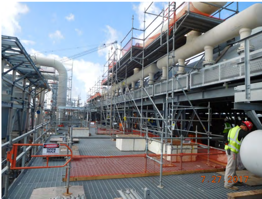
Train 5 – Cryo Rack - Air Cooled Exchanger Headers Installation
