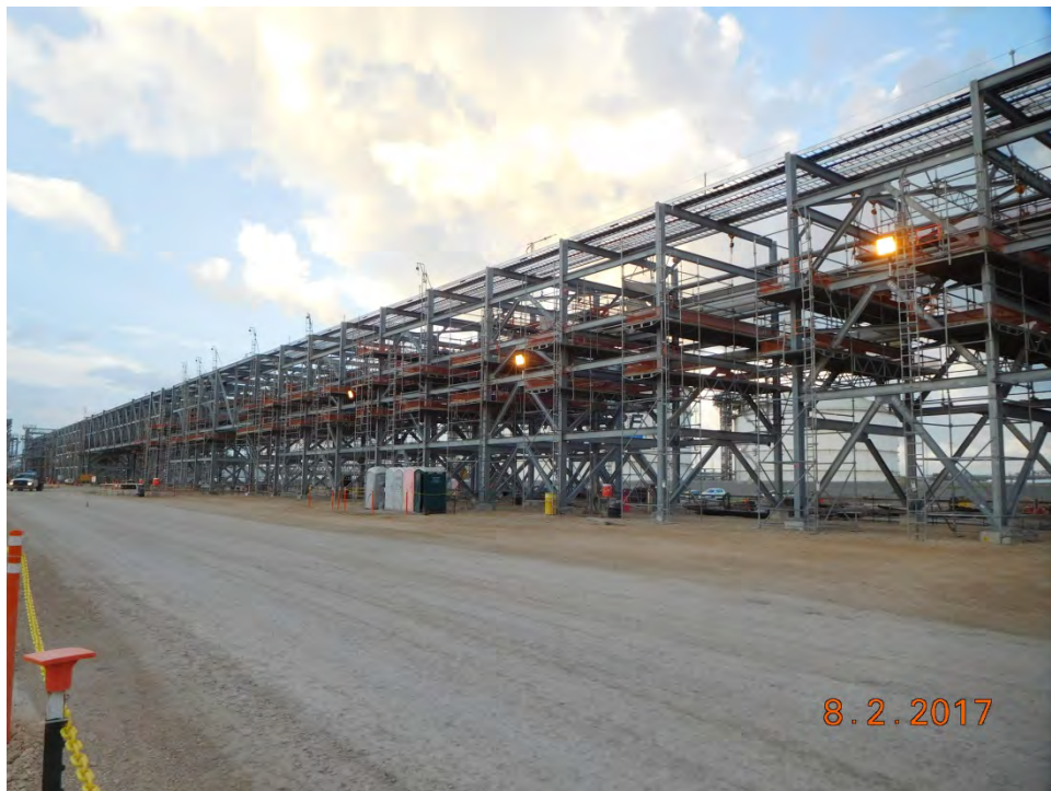
Stage 3 OSBL – Main North-South Pipe Rack
