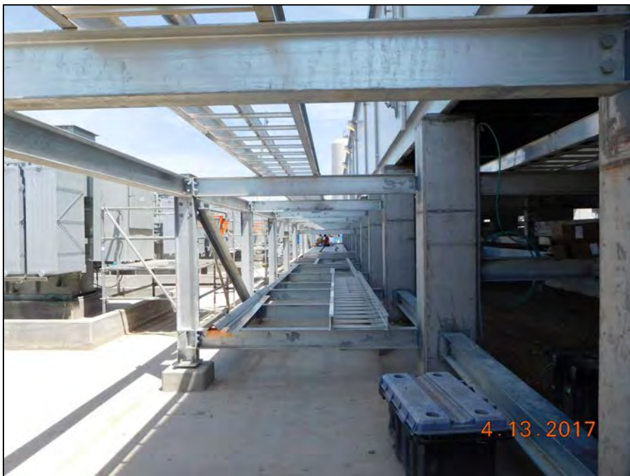
Stage 3 OSBL – Erecting Cable Tray on North Side of Utility Substation
