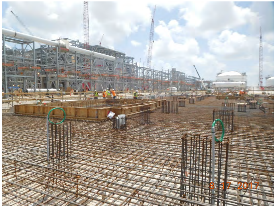
Stage 3 OSBL – Flare Modification Scope - Compressors Foundation
