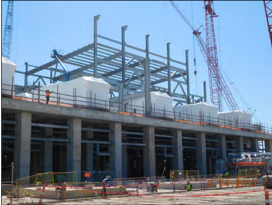
Train 5 – Structural Steel Erected Above A01 Compressors
