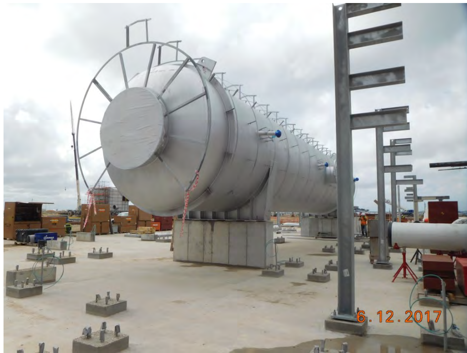
Train 5 – Thermal Oxidizer Installation
