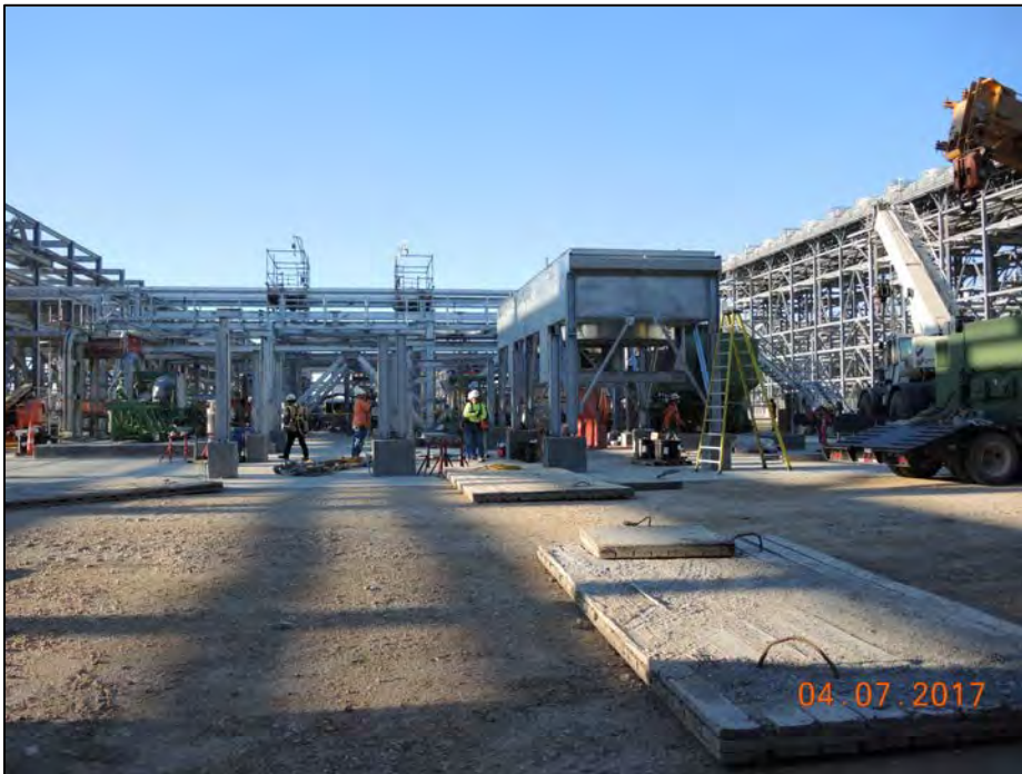
Stage 2 Flare Modification – Compressor Area
