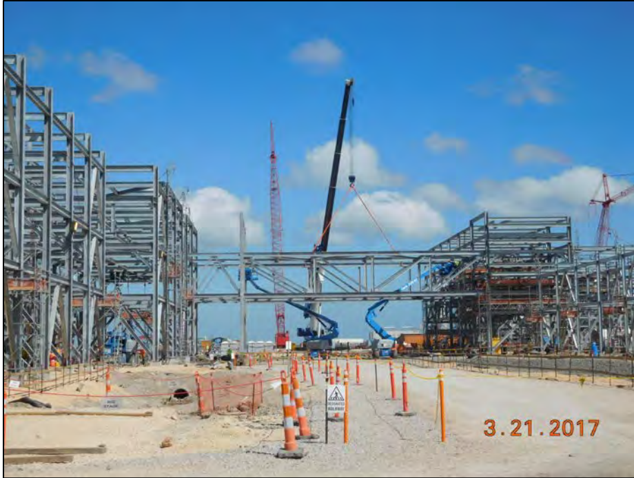
Stage 3 OSBL – Erecting Bridge Structure Across Primary Road
