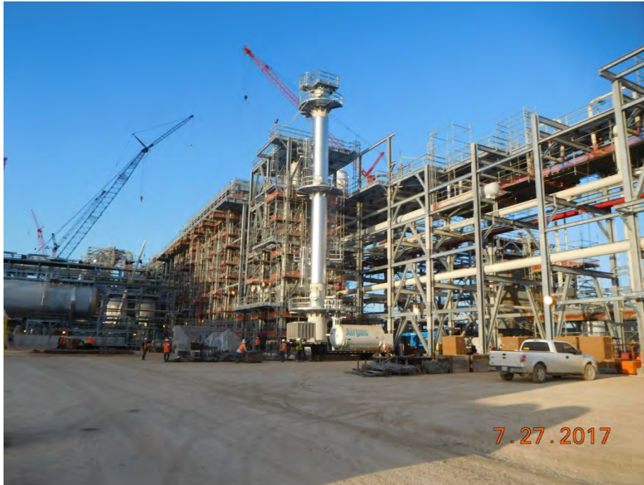
Train 5 – Southwest of ISBL - Condensate Stabilization and Utility Rack Areas
