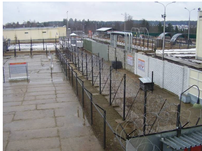
Figure 6. Example of a Nuclear Protective Force Training Facility
