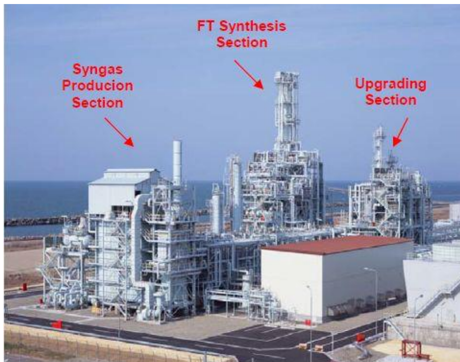
Japanese Gas to Liquids Pilot Plant, Niigata City, Japan
