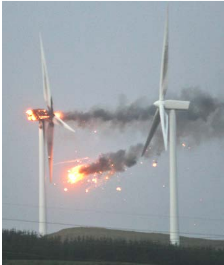
Wind turbine gearbox failure.
