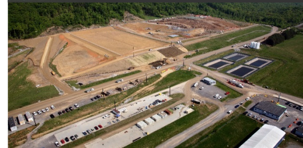
Current Onsite Disposal Facility
