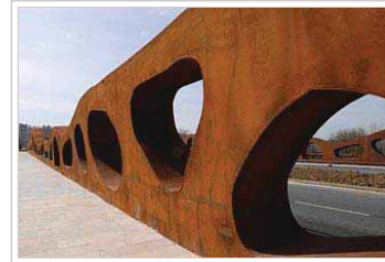
Abetxuko Bridge by J. Sobrino, PEDELTA, Abetxuko, Vitoria, Spain
