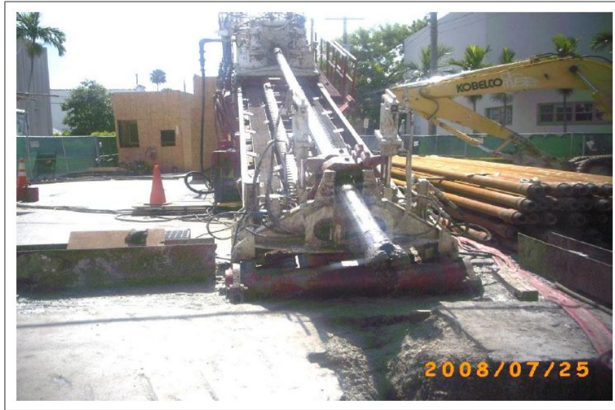
Figure 2-3. Underground Cable Installation – Horizontal Directional Drilling Equipment
