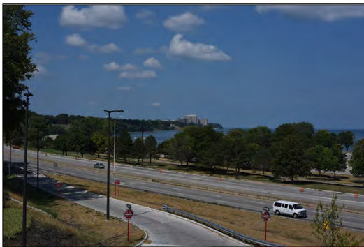
Inset 15 – Transportation LSZ - From Gordon Park overlooking East 72nd street
