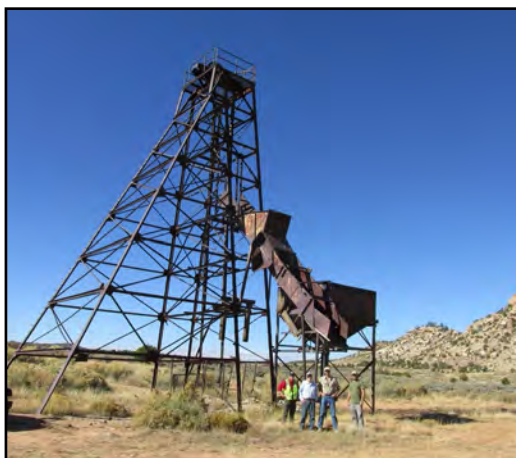
LP-16 shaft headframe in the Long Park area of BLM Uncompahgre Field Office, Montrose, County, Colorado.
