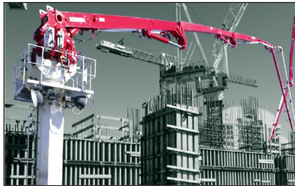
Slurry Placing Boom for Ritter Pile
