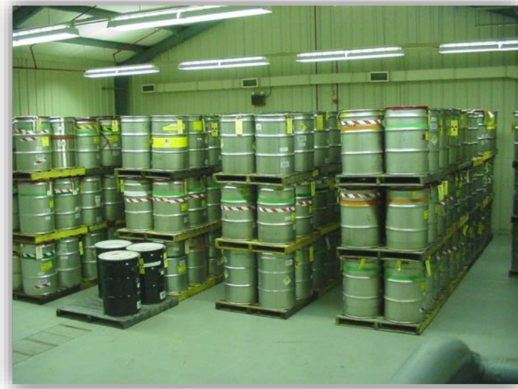
CH-TRU Waste Storage
