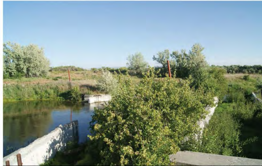
Photo 2. Looking south from the hatchery site toward the remnant concrete raceways.
