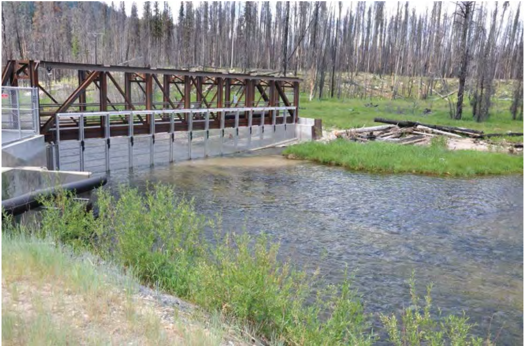
Figure 2-6b. Example of Bridge Weir in Operation (South Fork Salmon River Bridge Weir)
