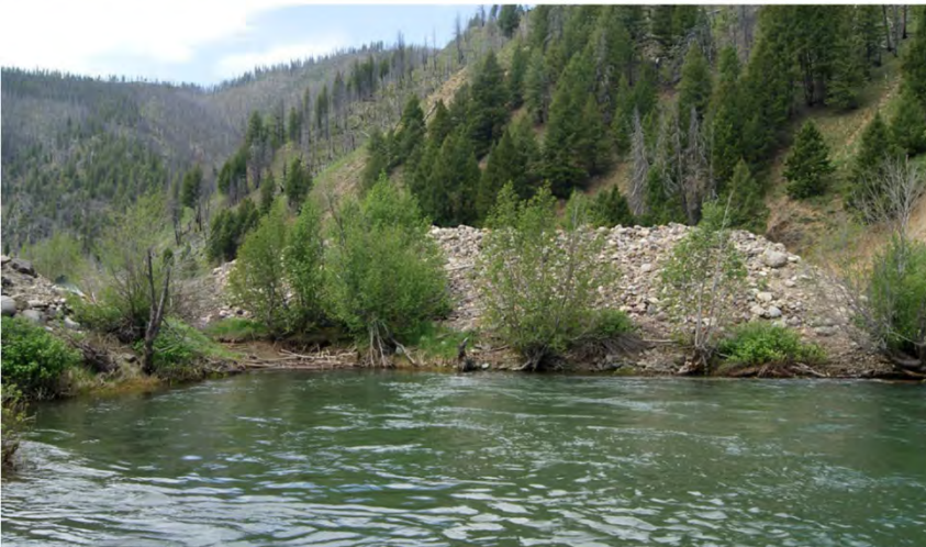
Photo 3. Looking southwest from an existing culvert outfall into the river toward the proposed satellite facility and existing dredge tailings.
