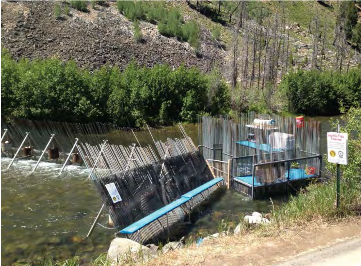
Figure 2-11. Example of a Temporary Weir Structure Proposed at the Yankee Fork and Panther Creek Weir Facilities under Alternative 2
