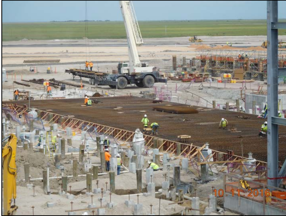
Train 5 - Acid Gas Removal Piperack Foundation
