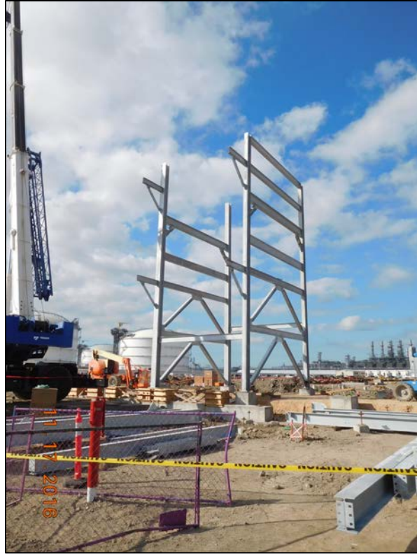
Stage 3 OSBL - First Steel Installed; in Main North-South Piperack (347R01)
