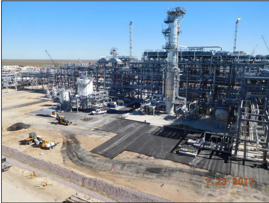
Train 3 – Asphalt Paving In Amine areas
