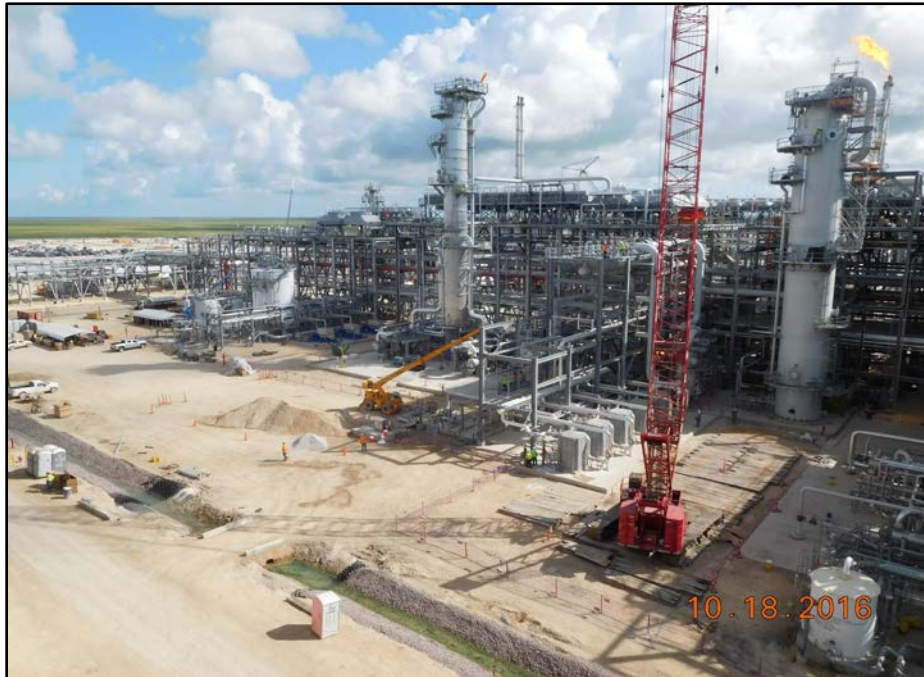
Train 3 - Amine Regeneration Area, Final Sump Prep in Progress
