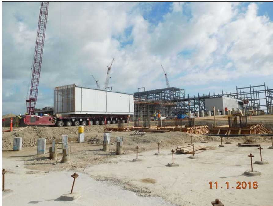
Train 5 - Compressor Substation Installation
