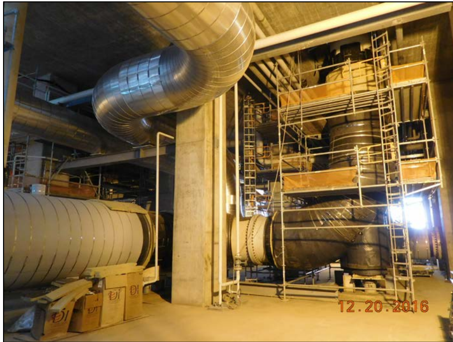
Train 4 - Insulation of Pipe Under Compressor Deck (1511 Compressors)
