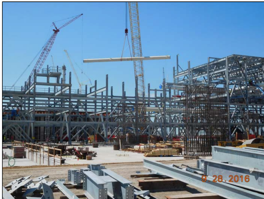
Train 5 - Flying Large Bore Pipe into Cryo Rack
