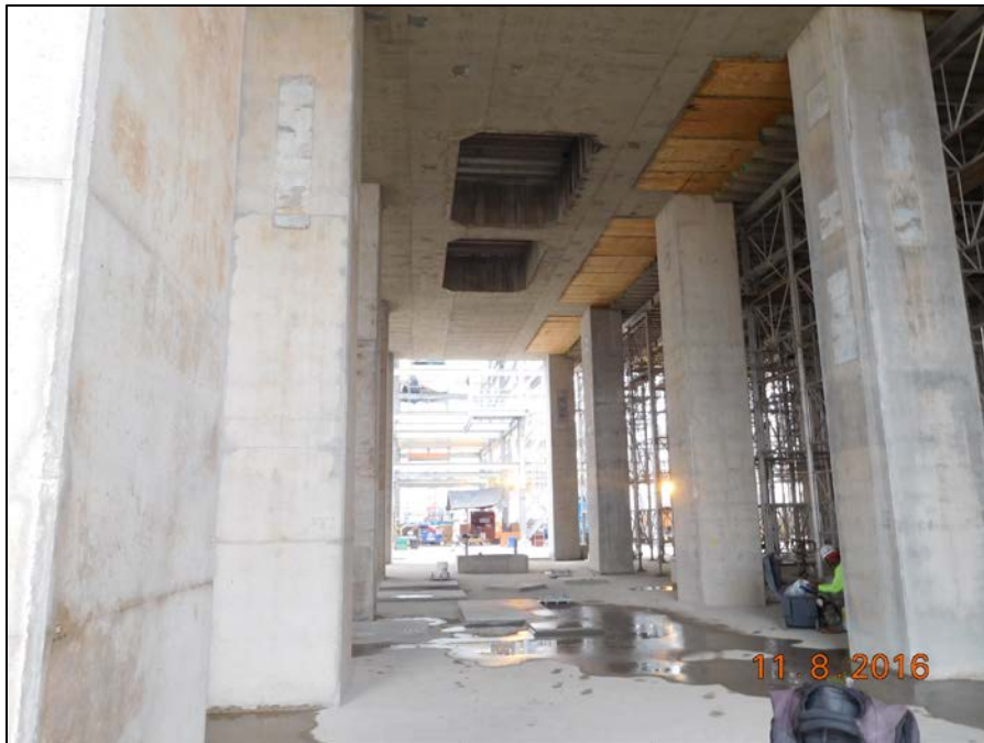
Train 5 - Compressor Area, Propane Deck Shoring Removed
