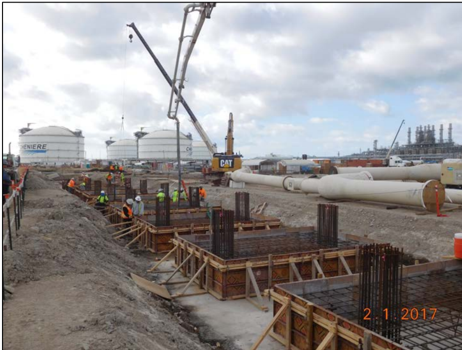
Stage 3 OSBL – Pouring Rack R06 Pile Caps Along N-S Run
