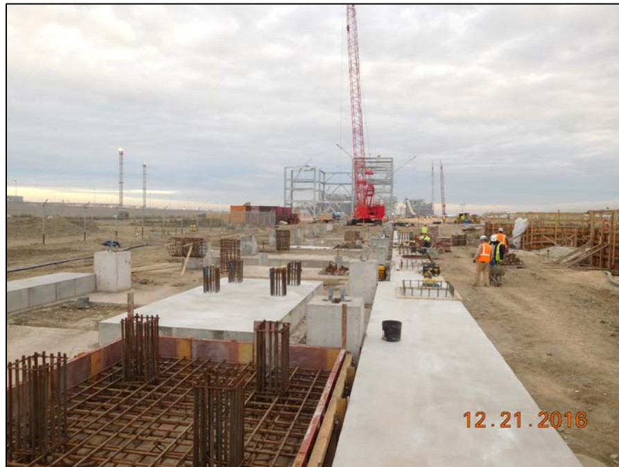
Stage 3 OSBL - Main North South Rack (347R01)
