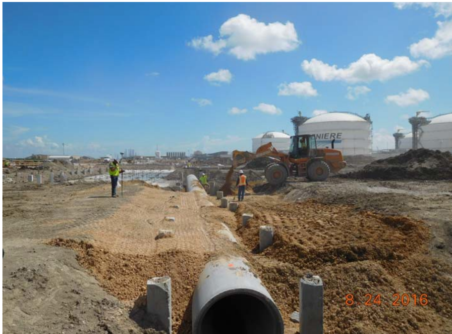
Stage 3 OSBL - Culvert Installation
