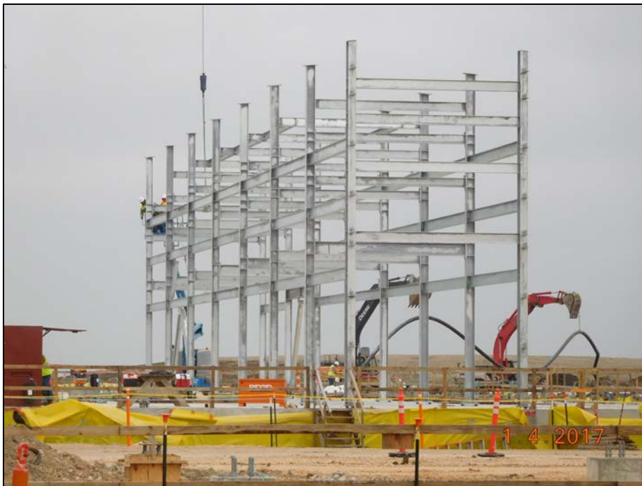
Stage 3 OSBL – Water Treatment Rack Steel Erection
