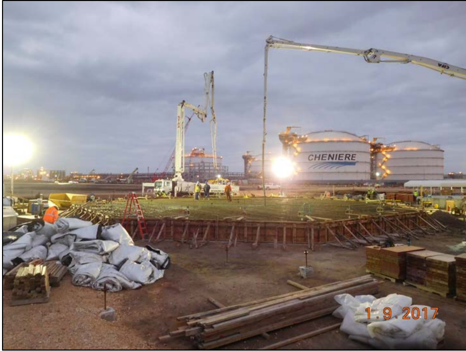
Stage 3 OSBL – Tank 30S-3603 Foundation Pour
