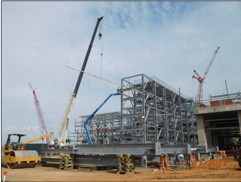
Train 5 – Loading Pipe in F01 Rack
