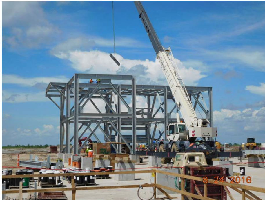
Train 5 - Commenced Installation of Steel in Propane Condenser Pipe Rack
