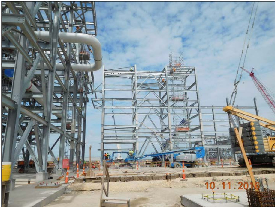
Train 5 - Mercury Removal Area Piperack Steel Erection
