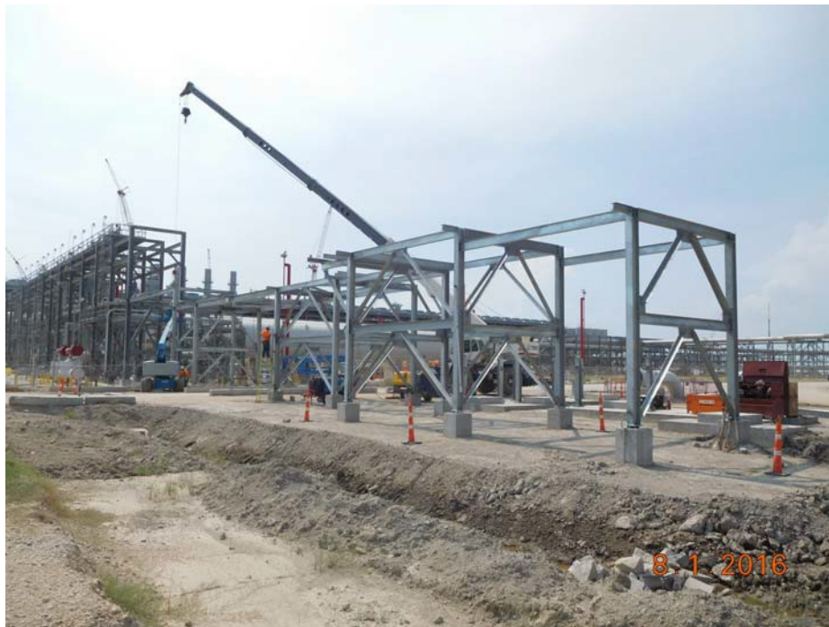
Stage 2 - East Metering Pipe Rack Installed
