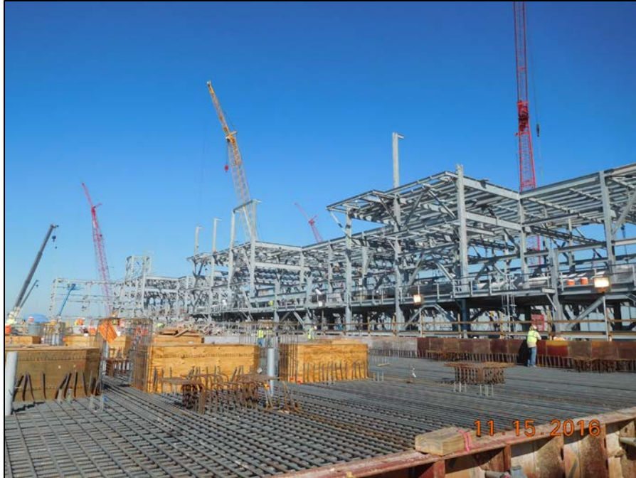
Train 5 - Form and Rebar Installation for Ethylene Deck in Compressor Area
