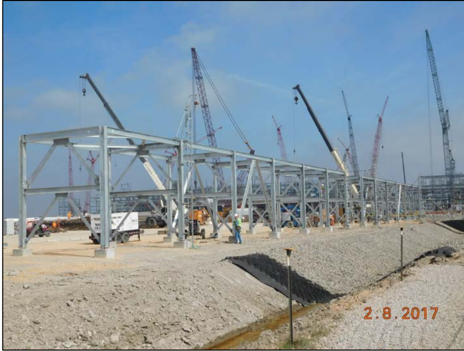
Stage 3 OSBL – 347R05 Steel Erection
