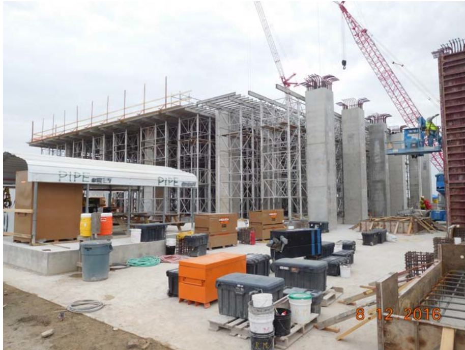
Train 5 - Installation of Shoring & Decking for Propane Deck
