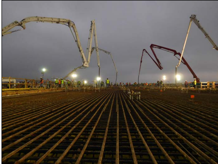
Stage 3 OSBL - Water Treatment Building Foundation Concrete Pour
