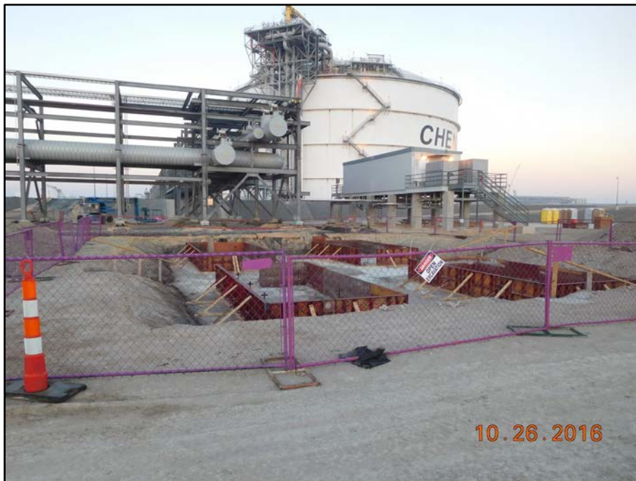
Stage 3 Revamp – North-South Piperack 326R01 Foundation Formwork
