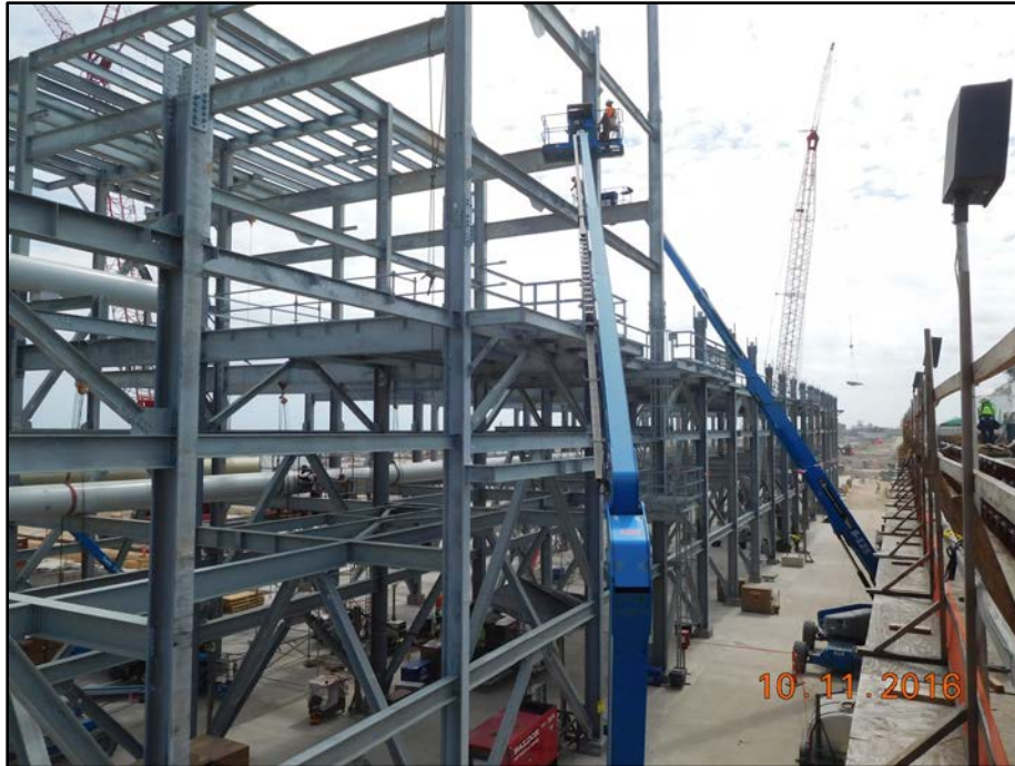
Train 5 - Cryo Rack Steel and Pipe Erection
