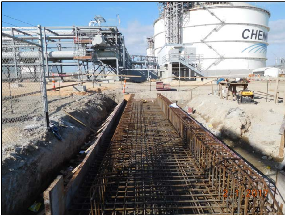
Train 5 – Revamp LNG Trench Rebar Near Tie-In Point In Existing Plant
