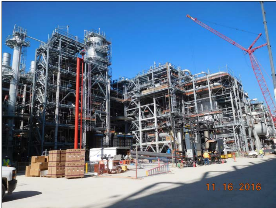
Train 3 – Setting Up to Fill Cold Boxes with Perlite
