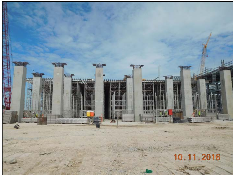
Train 5 - Last Compressor Deck Columns (Methane) Complete
