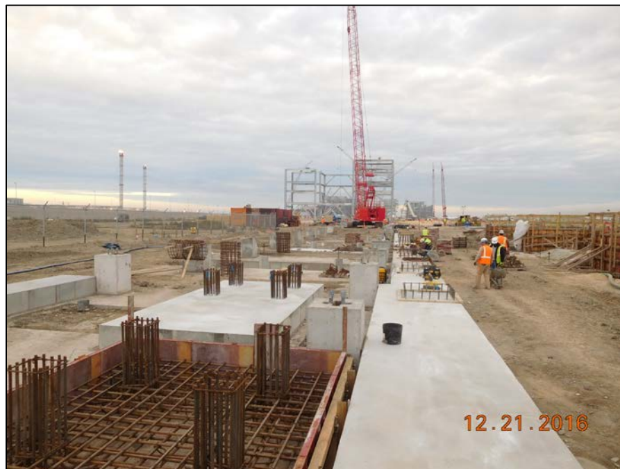
Stage 3 OSBL - Main North South Rack (347R01)
