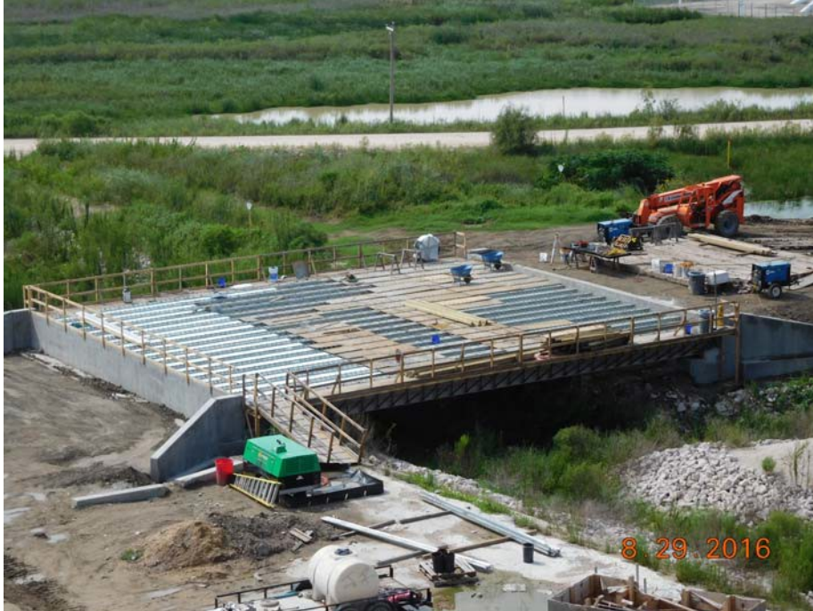
Stage 3 OSBL – Heavy Haul Road Bridge Installation
