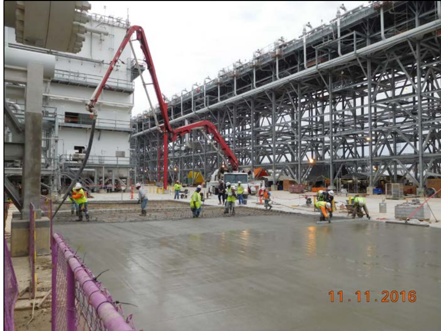
Train 3 - Area Paving
