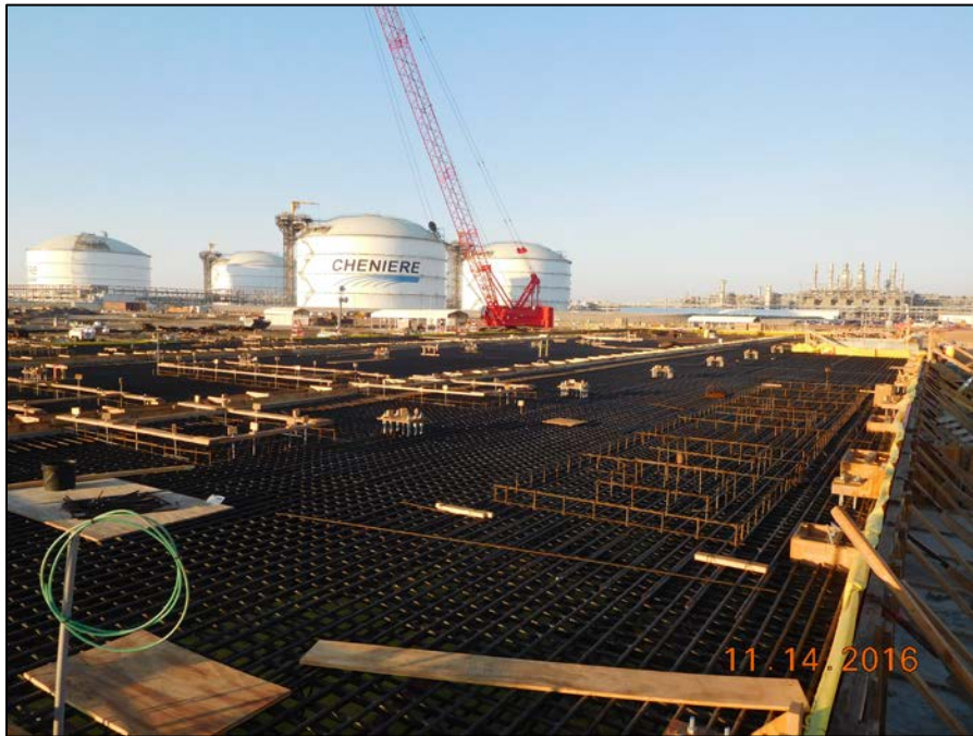
Stage 3 OSBL - Water Treatment Building Foundation
