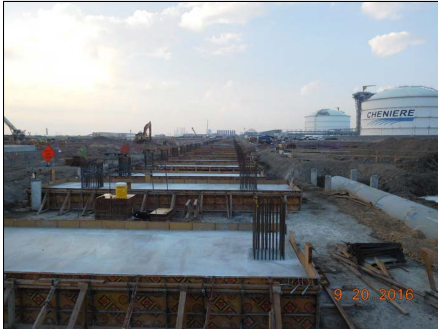
Stage 3 OSBL - Main North South Pipe Rack (R01) Foundations
