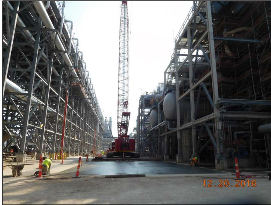
Train 3 - Area Paving of the Road Across Propane Refrigeration Area
