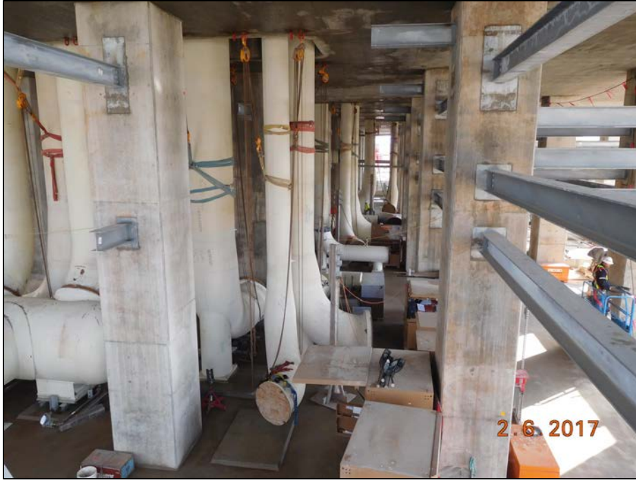
Train 5 – Hockey Stick Piping Installed
