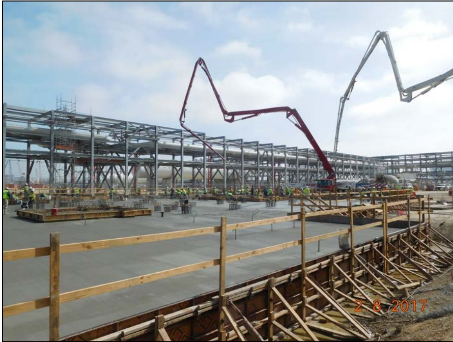
Stage 2 – Flare Modification Compressor Area
