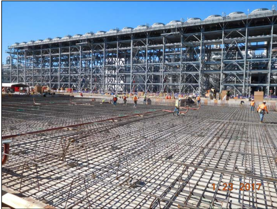
Stage 2 - Flare Modification Air Compressor Foundation In Progress
