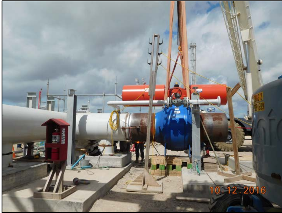
Stage 2 - East Metering Tie-in - Valve Installation
