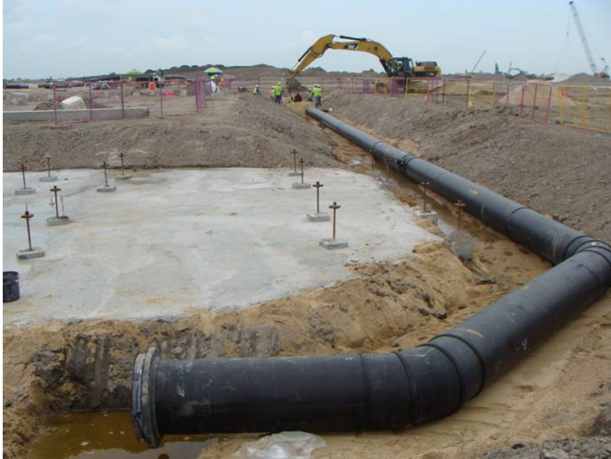
Stage 3 OSBL - Underground Firewater Pipe Installation
