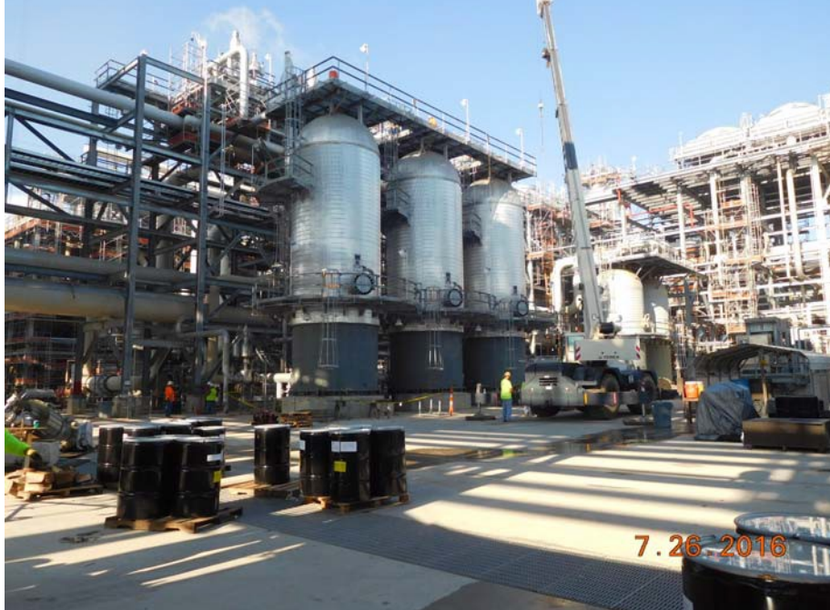
Train 3 - Installation of Internals in Molsieve Dehydration Vessels
