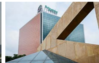
Schneider Offices, Bangalore
