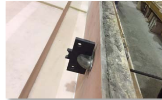
Installed carbon lifter at Gate precast
