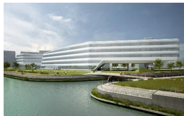
Johnson Controls Inc. (JCI) Asia-Pacific Headquarters (Shanghai China) – MPC open test-bed where industry and academia can develop and demonstrate their building control solutions.
