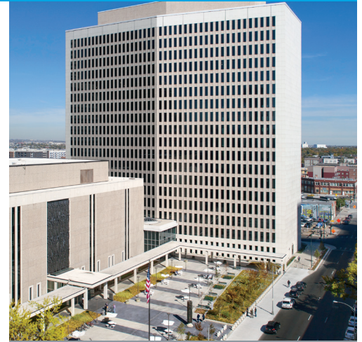
GSA replaced 3,300 troffer lights at the Byron G. Rogers federal building in downtown Denver to gain lighting energy savings of $49,200 annually. Photo courtesy of GSA
