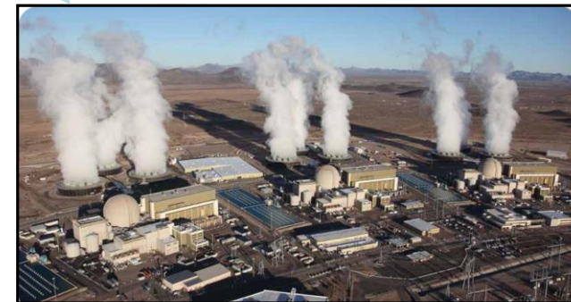
Palo Verde Nuclear Plant
