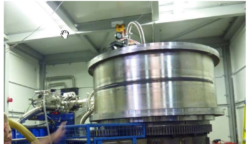
Thick section RPEB weld. Courtesy of TWI
