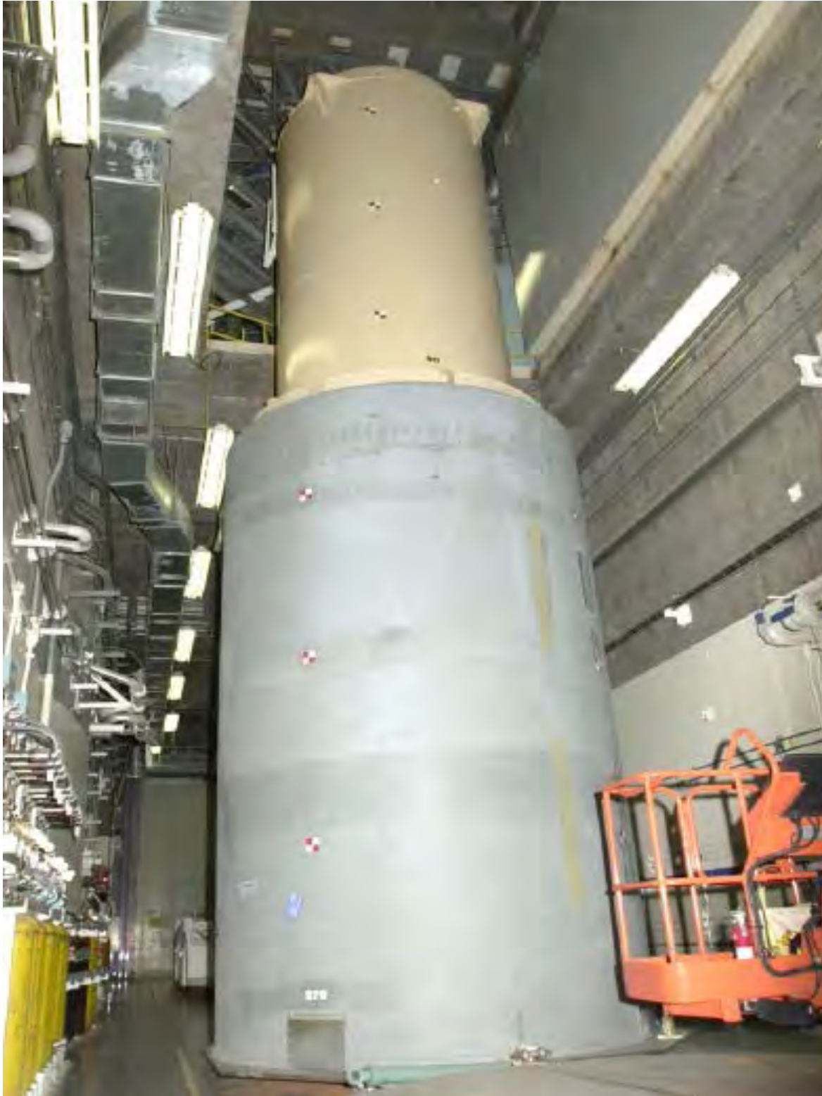
Figure 4-4 Holtec International HI-STORM “Stack-up” Vertical Canister Transfer
