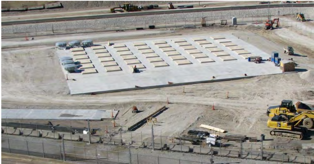
Holtec HI-STORM UMAX, Completed Pad Construction, Callaway ISFSI
