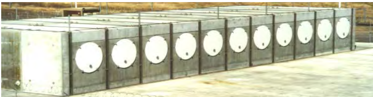
Figure 3-4 Horizontal Storage Modules at the Rancho Seco Plant
