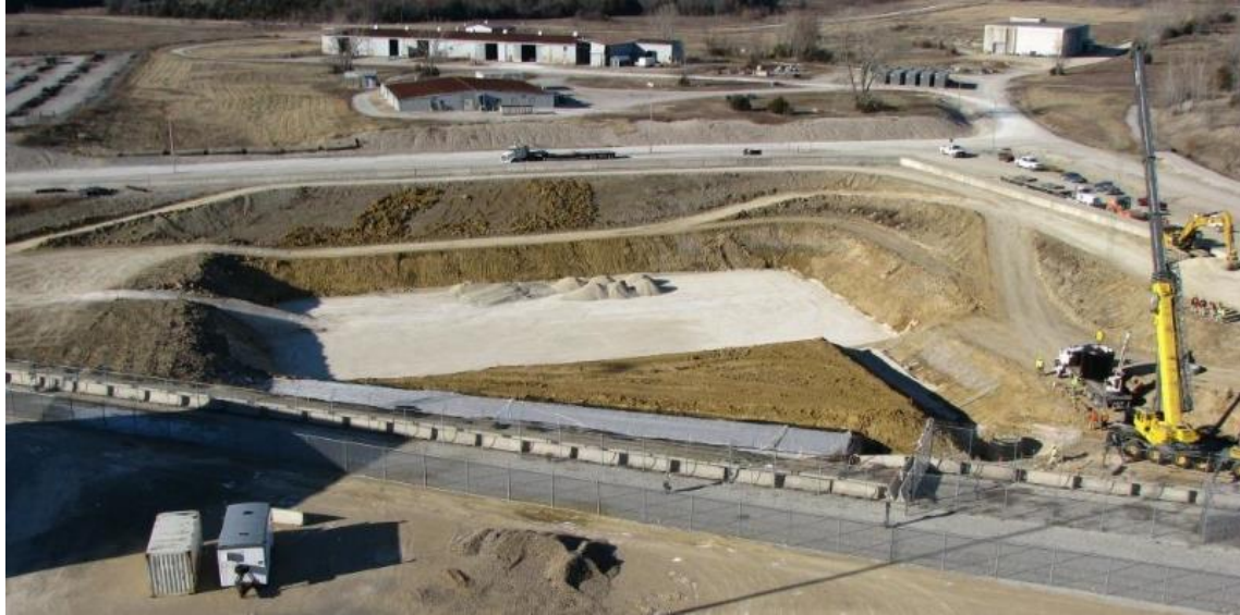
Figure 4-15. Excavation Activities at Callaway Nuclear Site
