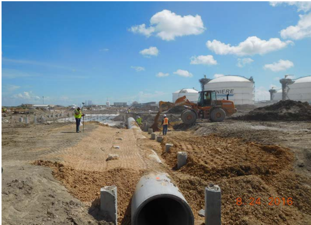
Stage 3 OSBL – Culvert Installation
