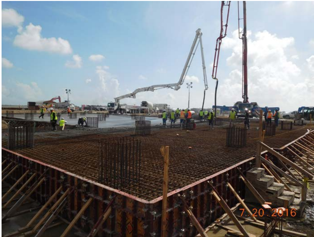
Train 5 – First Concrete Pour of Propane Condenser Pipe Rack Foundation
