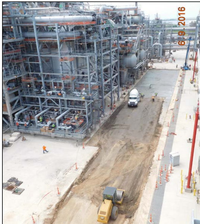
Train 2 - Area Paving of the Road Inside ISBL
