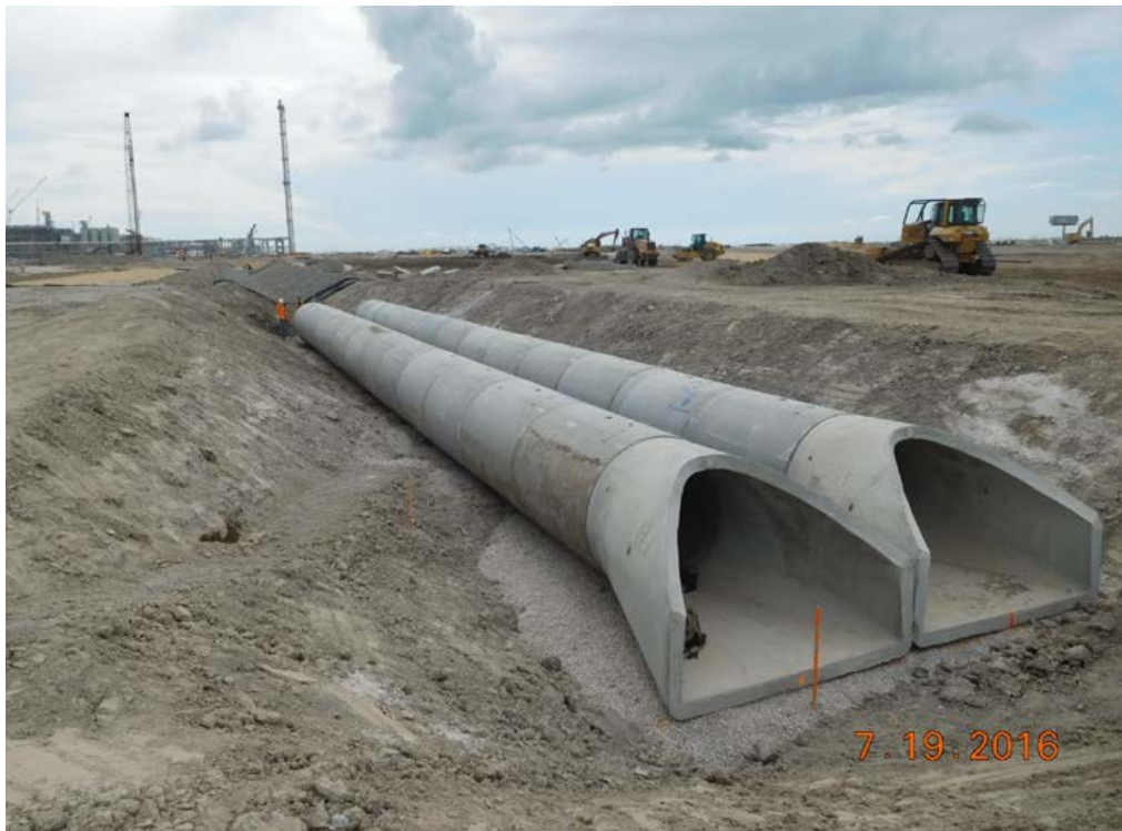
Stage 3 OSBL – Culverts, Heavy Haul Road (Northeast of ISBL)
