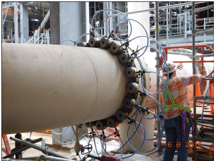
Train 3 - Hydraulic Bolt Tensioning
