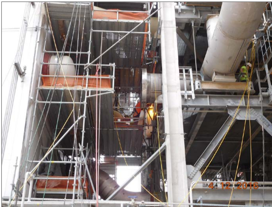
Train 2 - Installation of Aboveground Pipe Connections to Ethylene Cold Box
