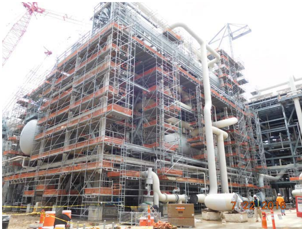
Train 3 – Propane Refrigeration Area, the All-Structure Multi-Discipline Scaffolding is Erected
