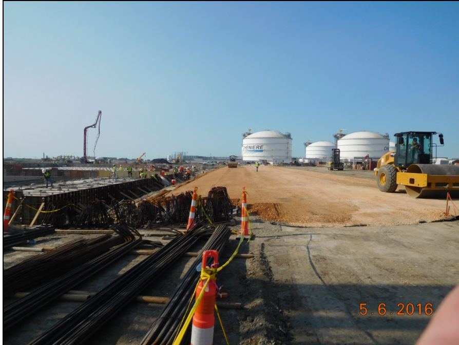
Train 5 - Installation of Primary Road #4 (West of ISBL)
