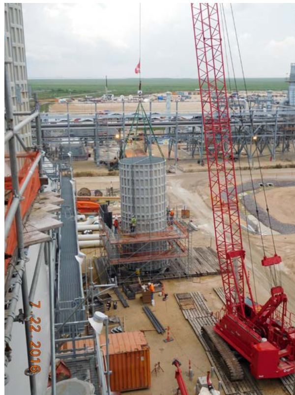
Train 4 – Subcooler Stacks Erection in Progress
