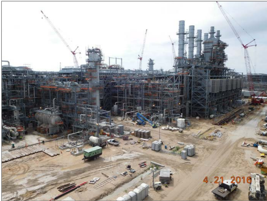
Train 3 - Overview from North West
