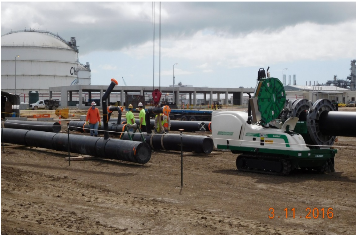
Train 5 – Underground Firewater Pipe Assembly
