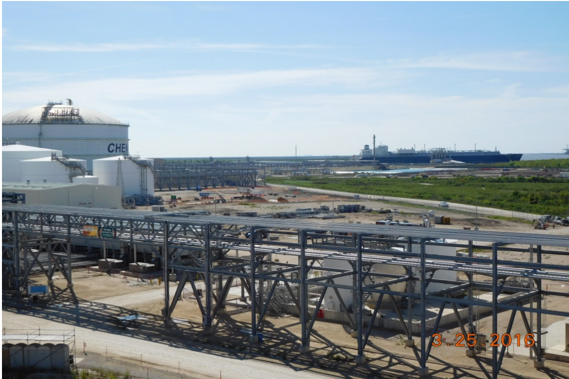
Train 1 –LNG commissioning cargo being loaded into the LNG Carrier.
