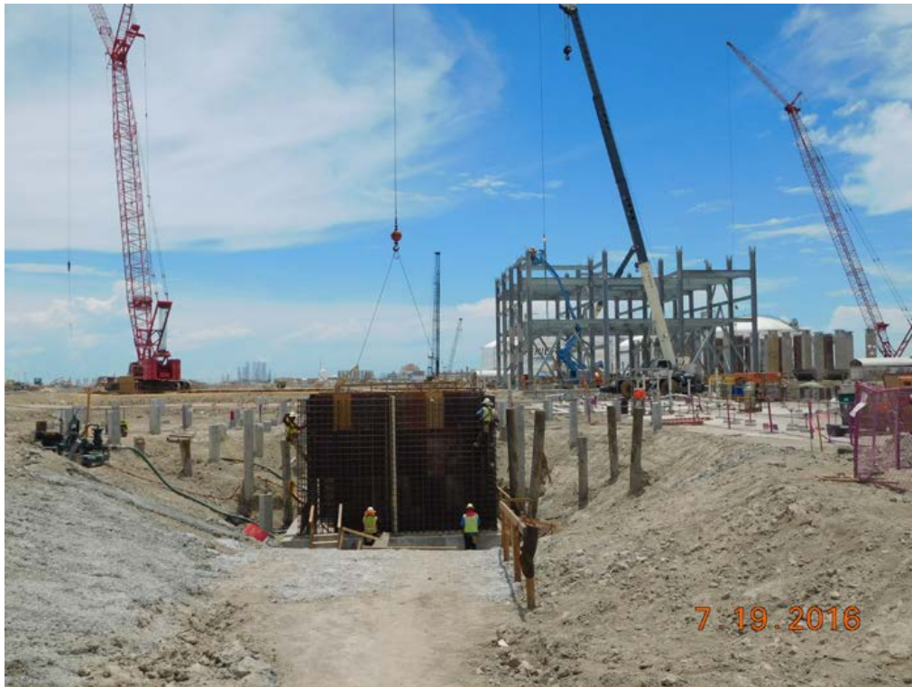
Train 5 – Hot Oil Sump Wall Installation
