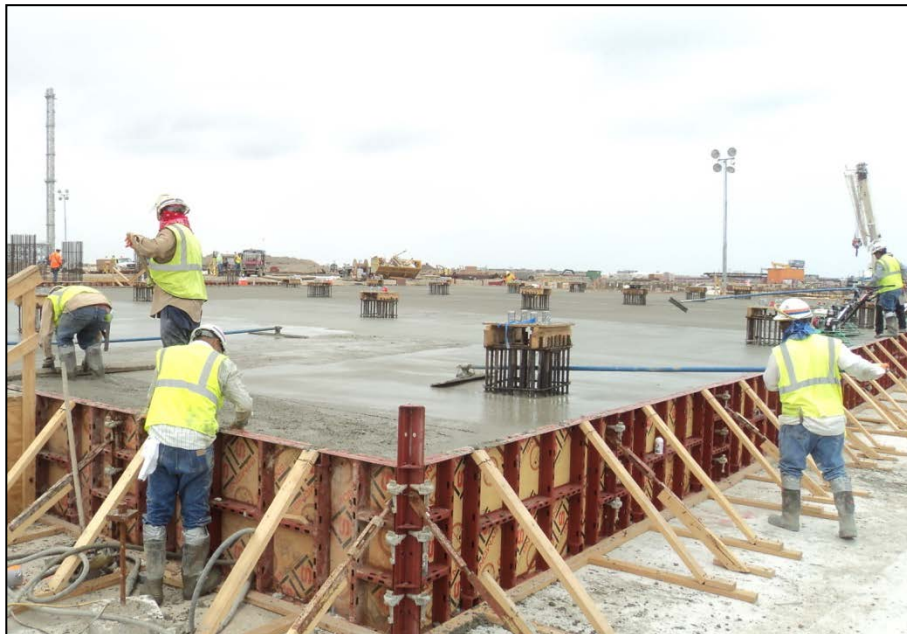
Train 5 - Concrete Pour of Section 5 of the Cryo Rack
