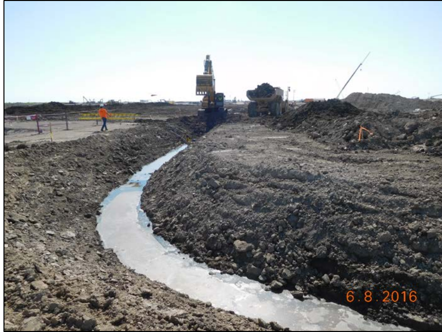
Stage 3 OSBL - Excavation for Trench Installation (OSBL1 Trench A North End)
