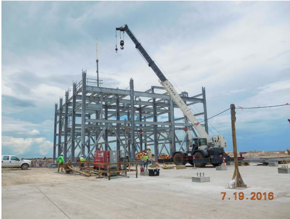
Train 5 – Commenced ISBL Steel Erection, Cryo Pipe Rack Area
