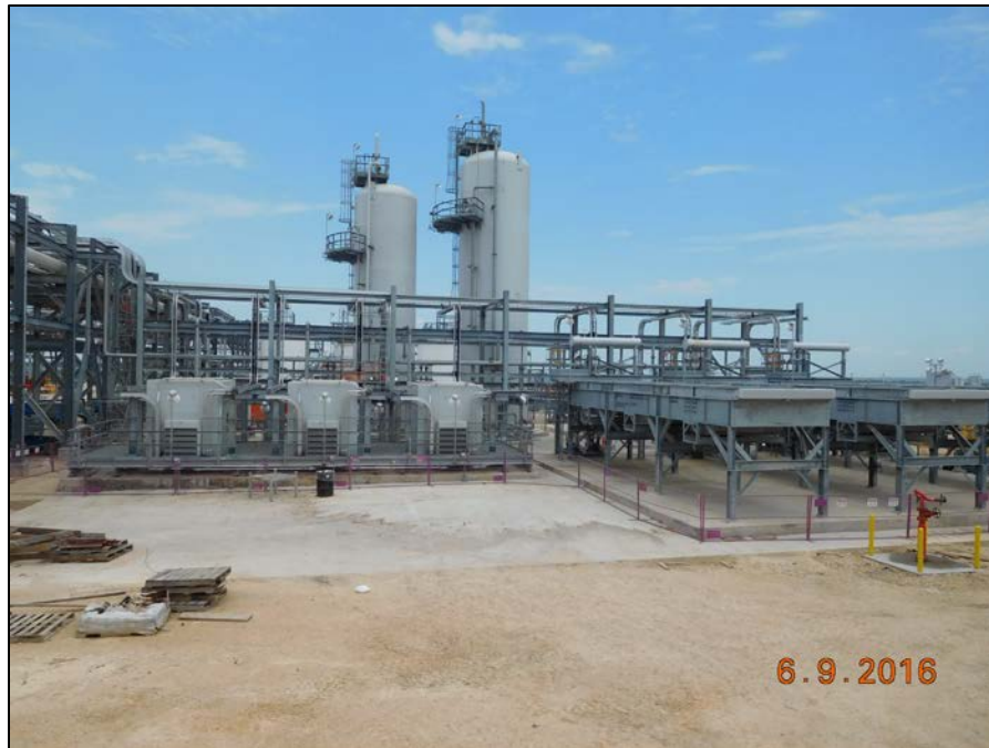
Stage 2 OSBL - Air Compressors Commissioned
