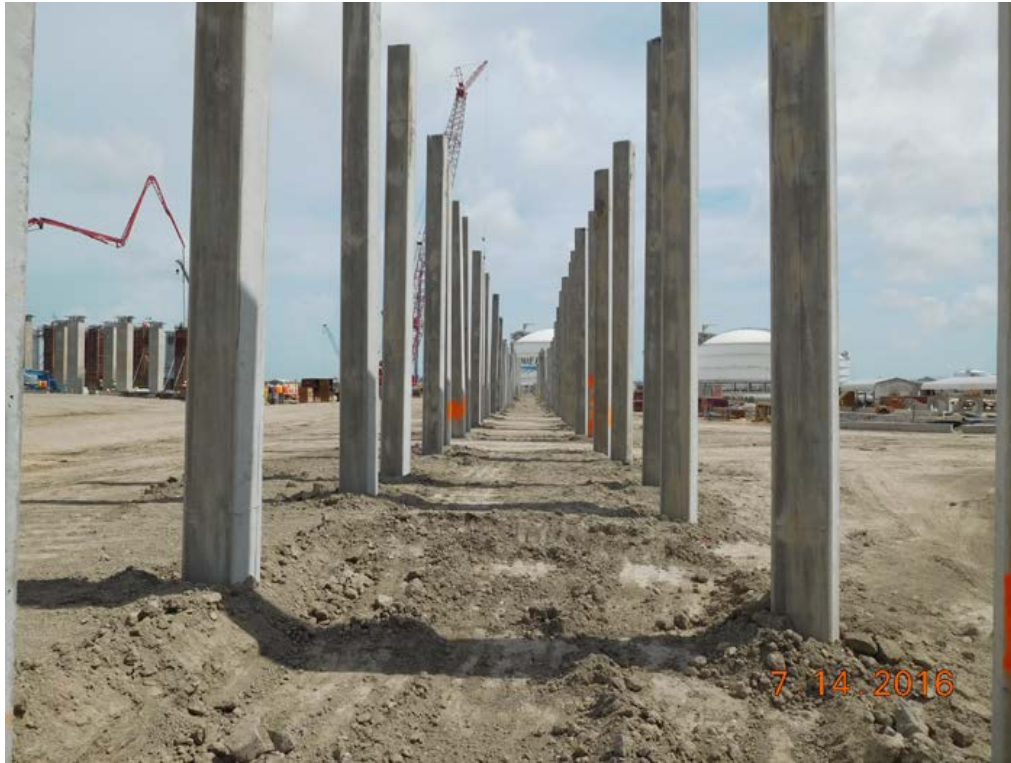
Stage 3 OSBL – Piling, Pipe Rack R06 Area
