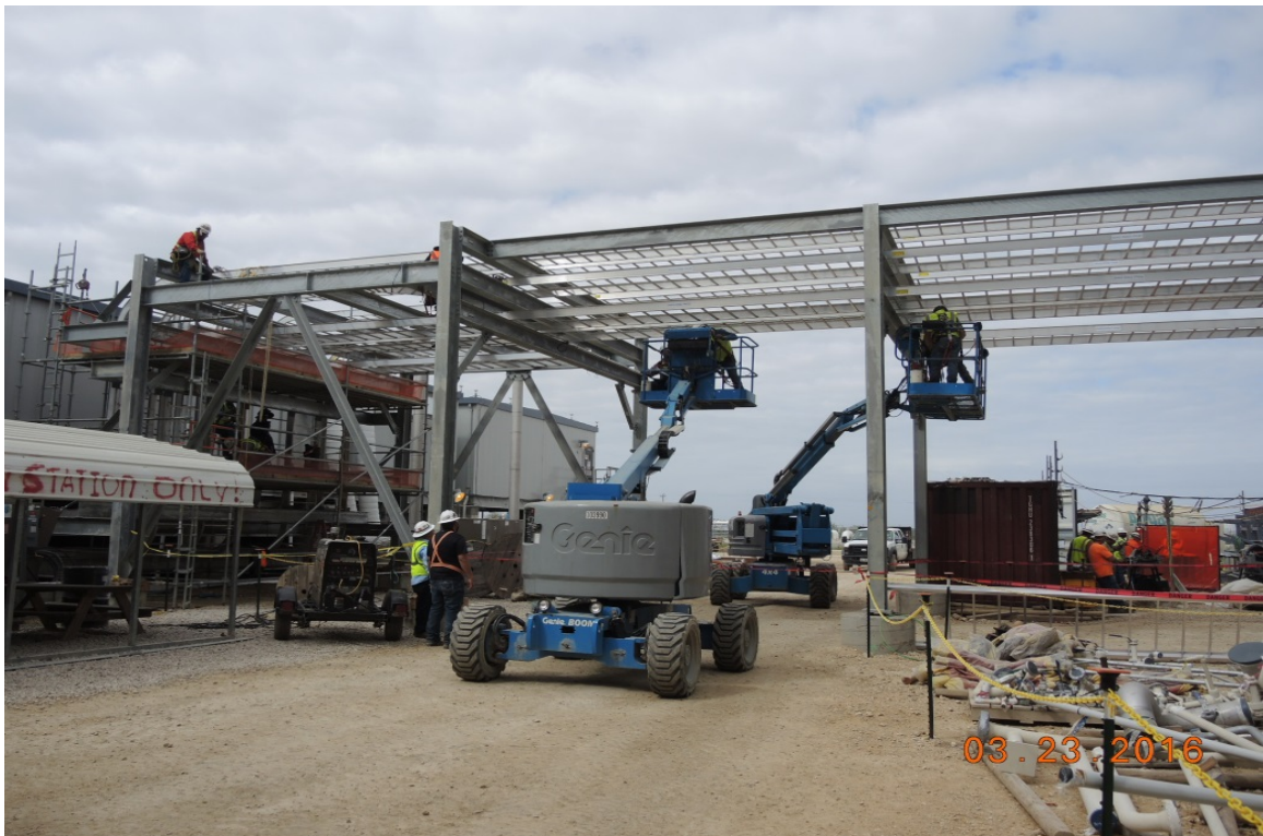
Train 4 – Cable Tray Installation from Compressor Substation to Compressor Deck
