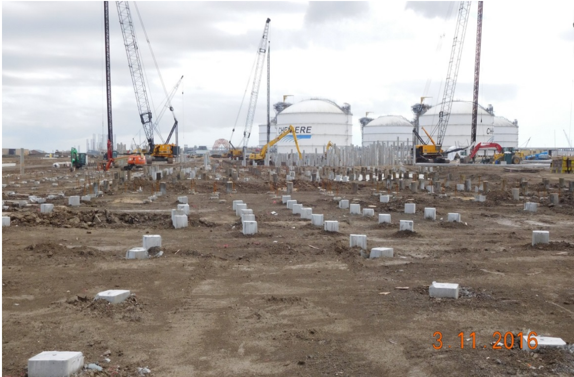
Train 5 – Piling in ISBL
