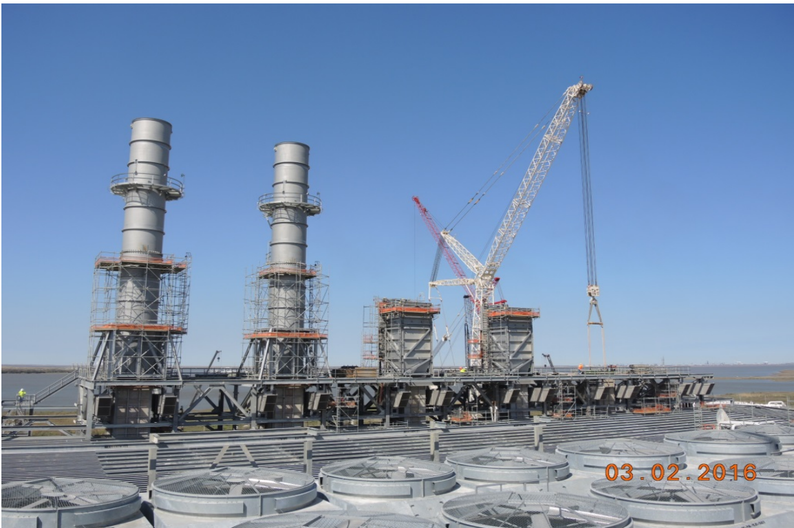
Train 4 – Turbine Exhaust Stack Installation in Compressor Area
