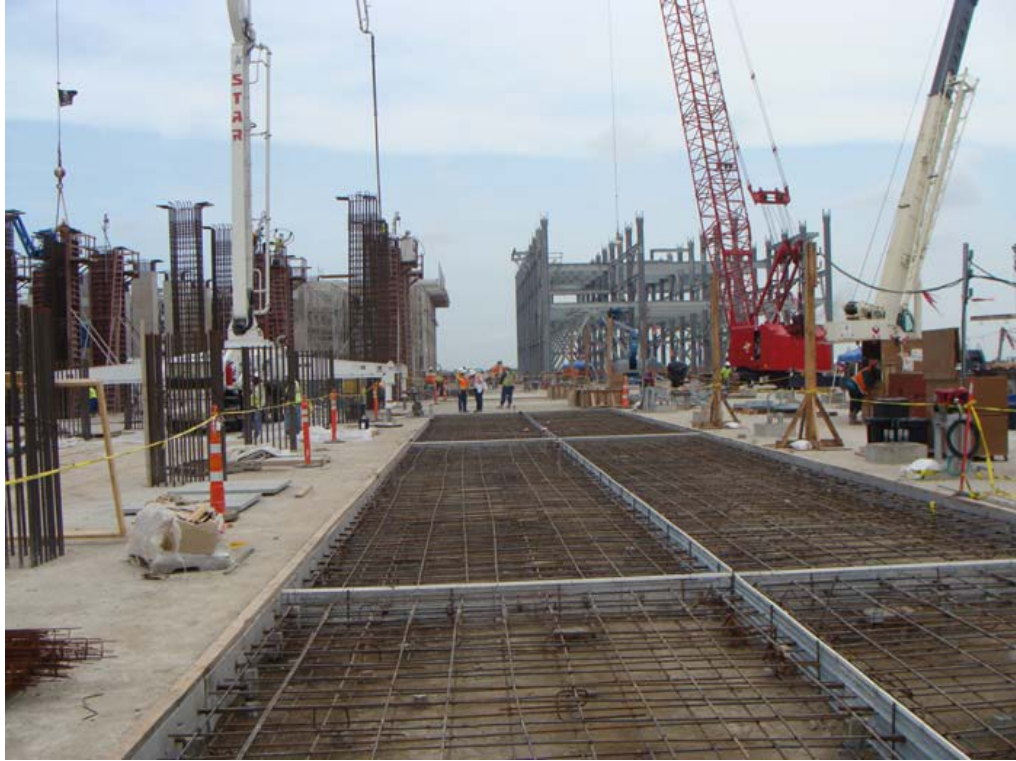
Train 5 – Area Paving between Compressor and Cryo Rack Areas
