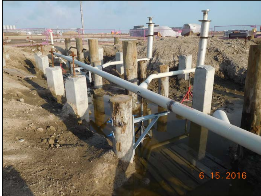
Train 5 - Amine Underground Pipe Installation in Amine Storage Area (ISBL)
