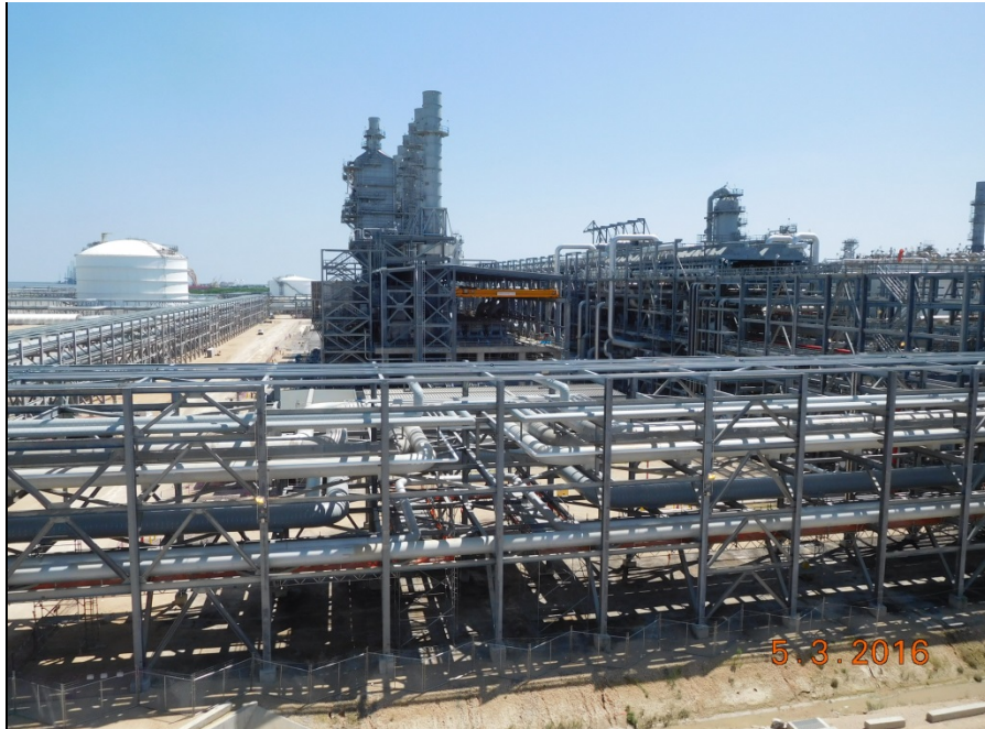
Train 1 - View from North; Area Security Fences Are Installed
