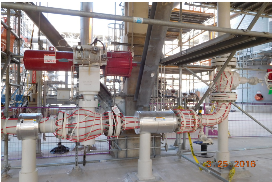
Train 2 – Electrical Heat Tracing Installation in Cryo Rack Area
