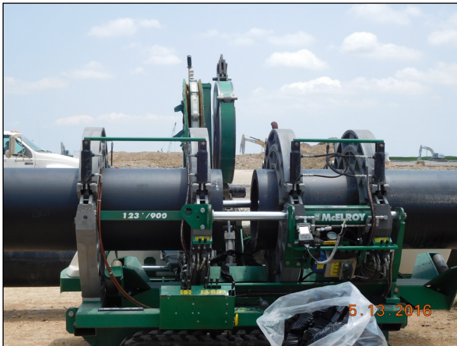
Train 5 - Underground Firewater HDPE Pipe Fusion
