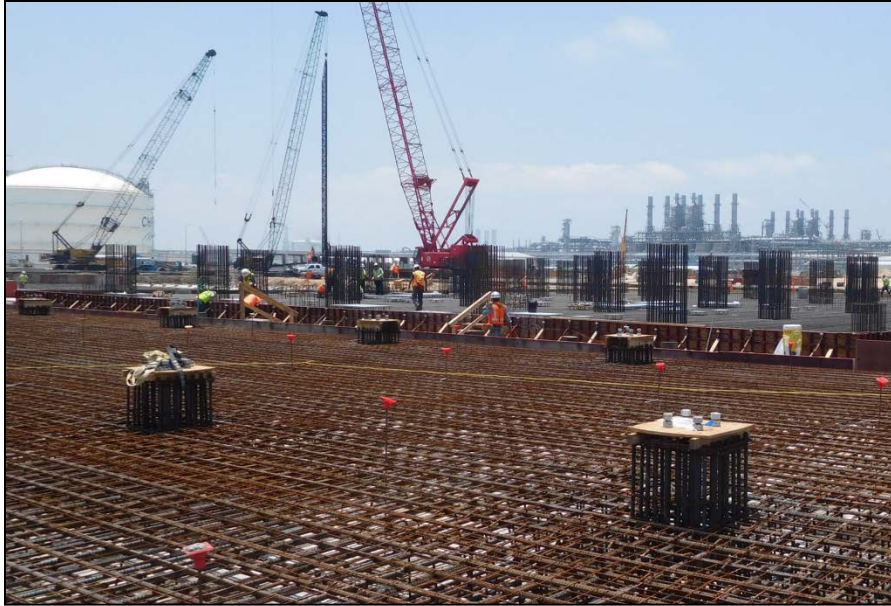
Train 5 – Cryo Rack (Front) and Compressor Area (Back) Foundation Preparation
