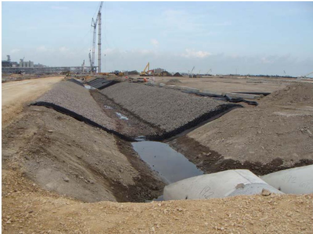
Stage 3 OSBL – Drainage Ditch Installation
