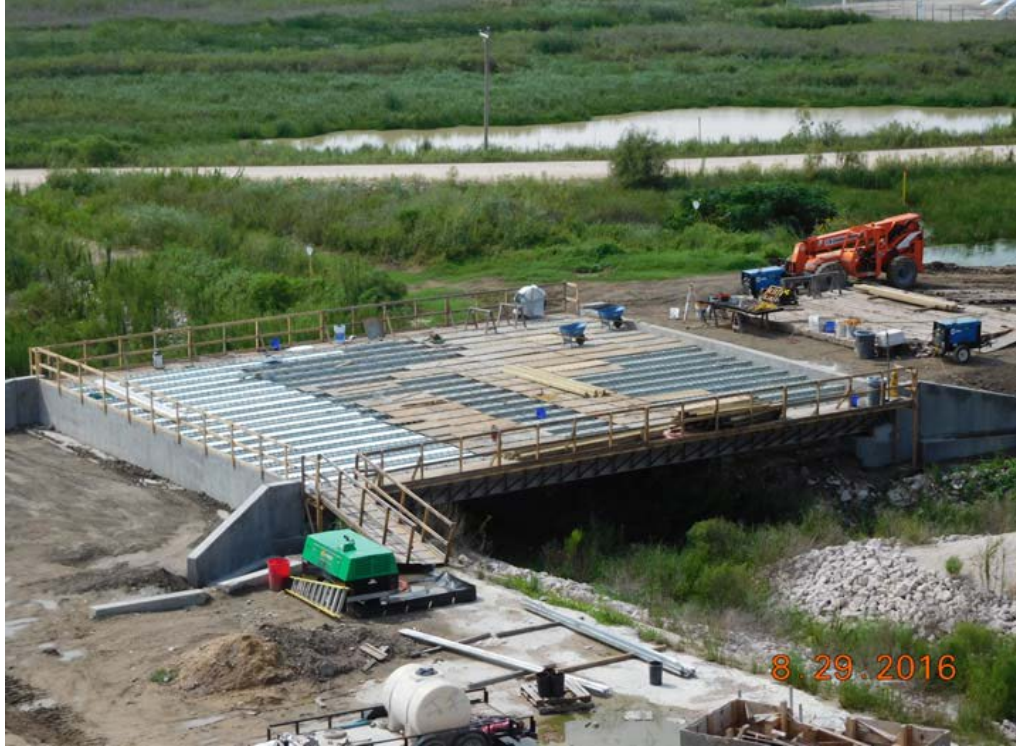
Stage 3 OSBL – Heavy Haul Road Bridge Installation
