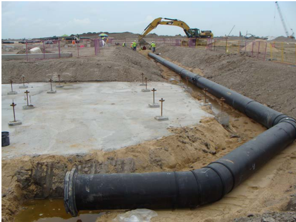
Stage 3 OSBL – Underground Firewater Pipe Installation
