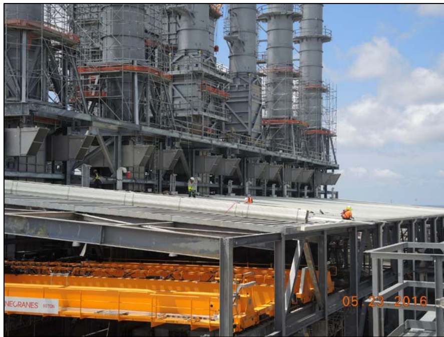
Train 4 - Compressor Area Roofing Installation
