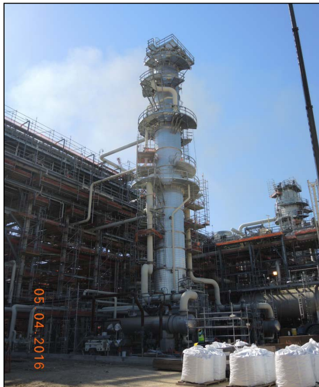
Train 3 - Installation of Catalysts (Nutter Rings) in Solvent Regeneration
