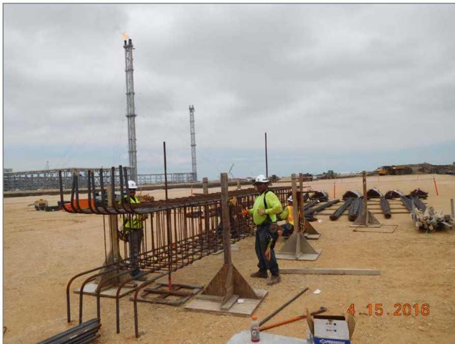
Train 5 - Prefabricating Rebar for Compressor Deck Columns
