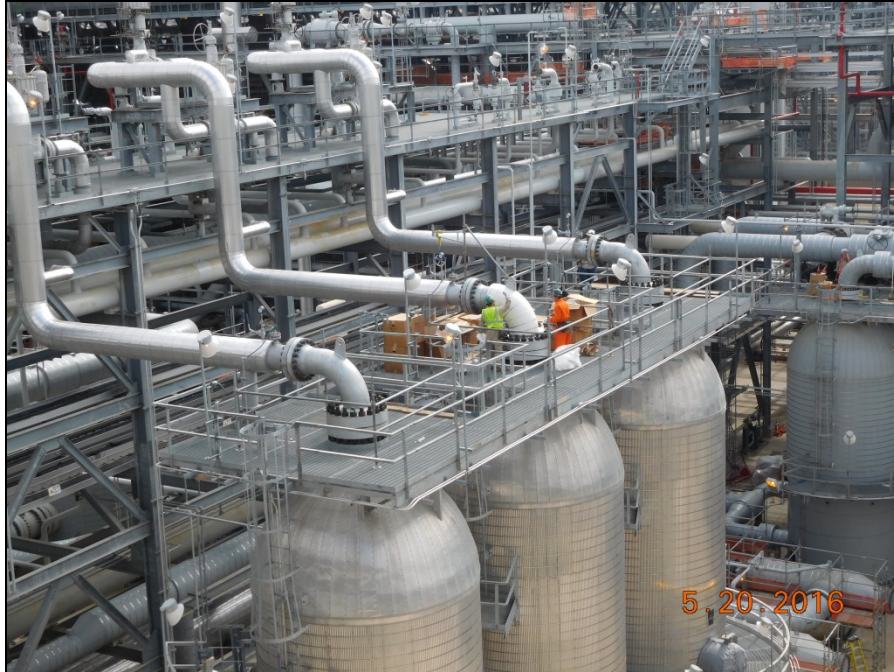
Train 2 - Insulation of Pipe on Top of Mole sieve Dehydration Vessels
