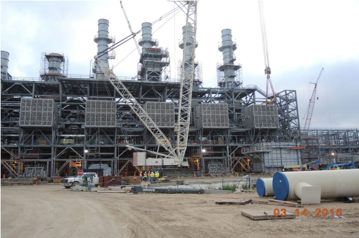
Train 4 – Lifting the WHR Unit in Compressor Area
