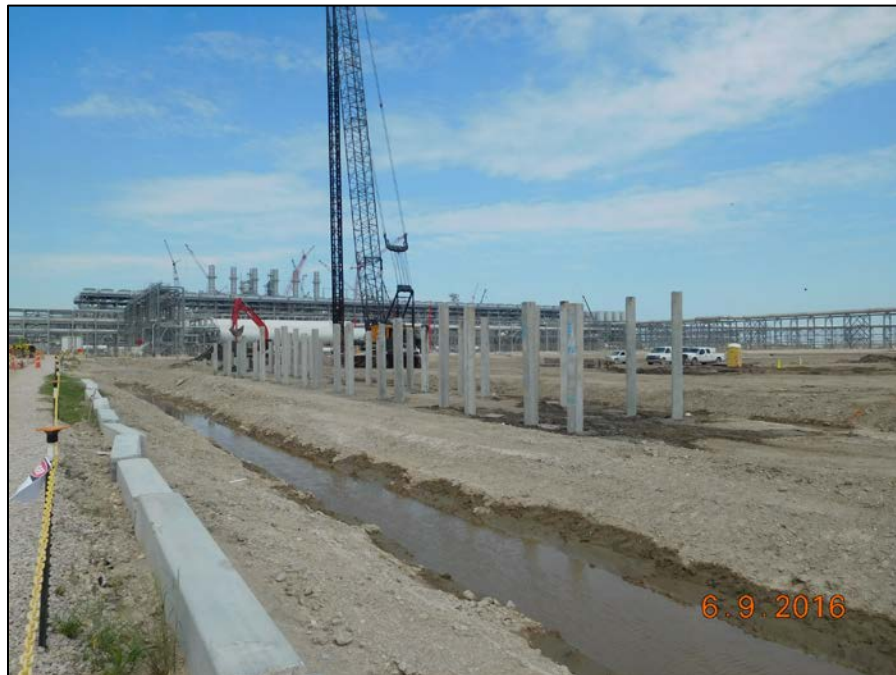
Stage 3 OSBL - Piling of Propane Refrigerant Storage Area Pipe Rack (347R05)
