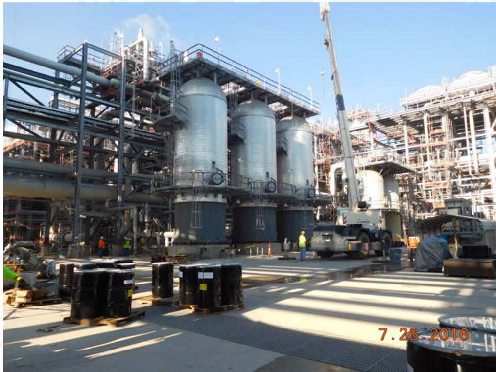
Train 3 – Installation of Internals in Mole Sieve Dehydration Vessels
