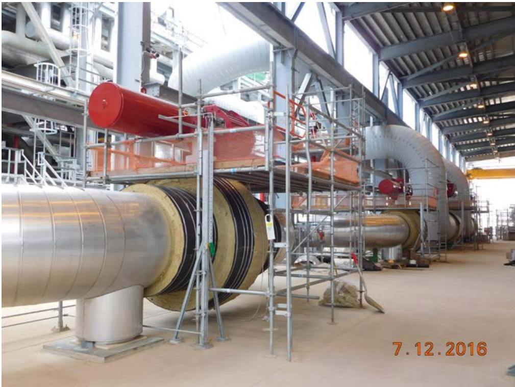
Train 2 – Cold Insulation Installation on Pipe Flanges on Compressor Deck
