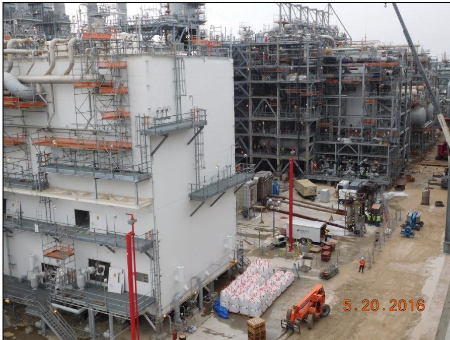
Train 2 - Installation of Perlite in Cold Boxes
