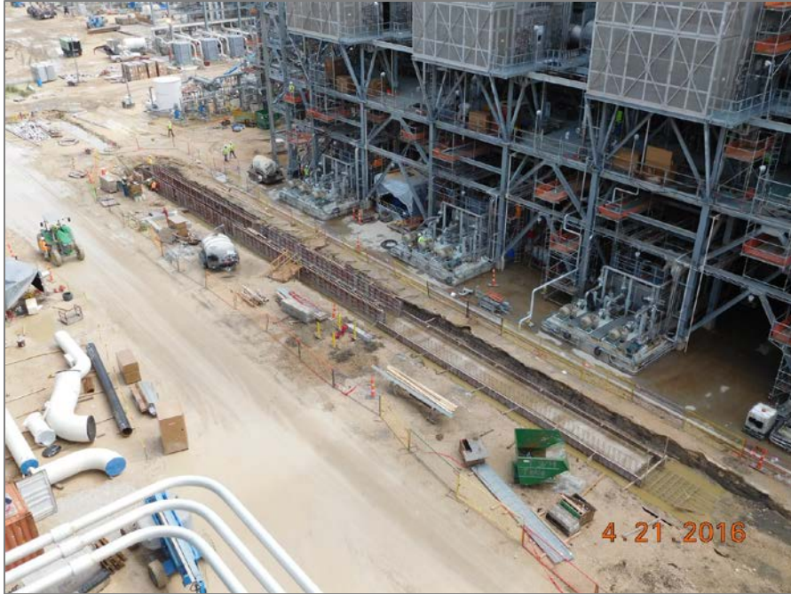
Train 3 - Installation of Oil Spill Trench in Compressor Area
