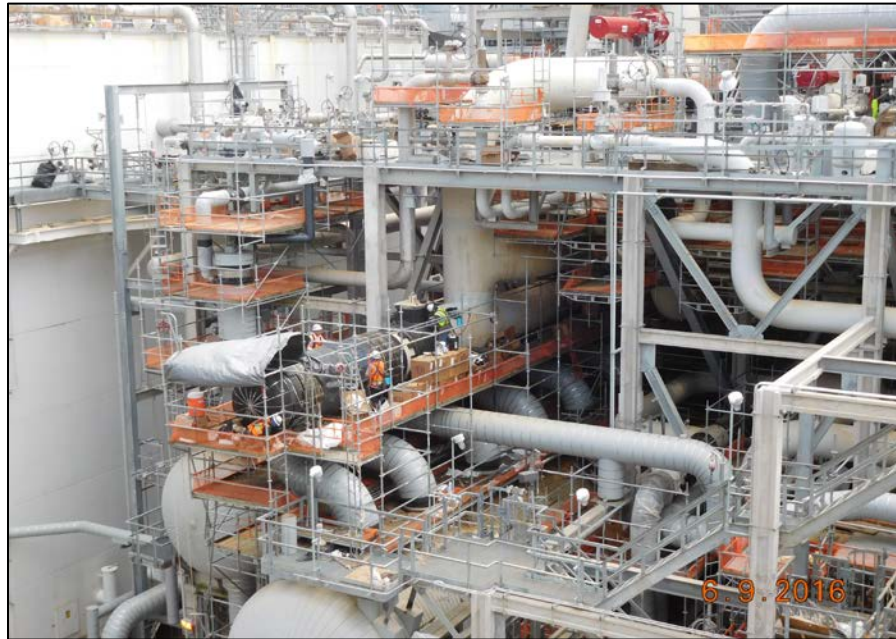
Train 2 - Pipe Insulation Installation in Propane Refrigeration Area
