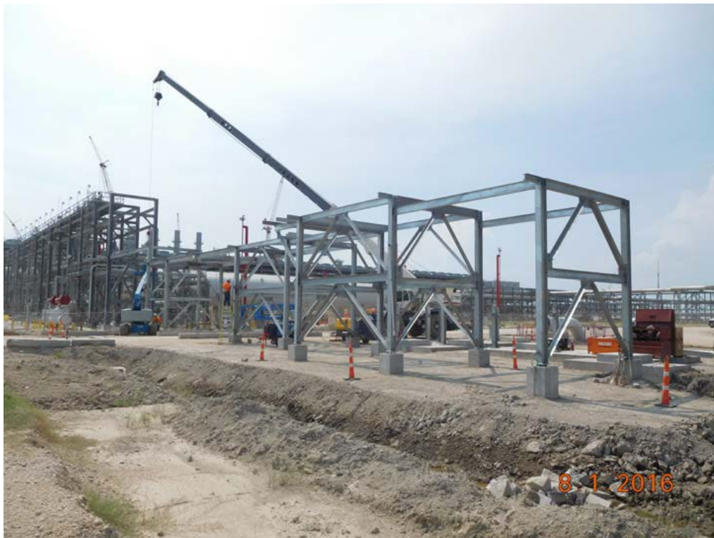
Stage 2 – East Metering Pipe Rack Installed
