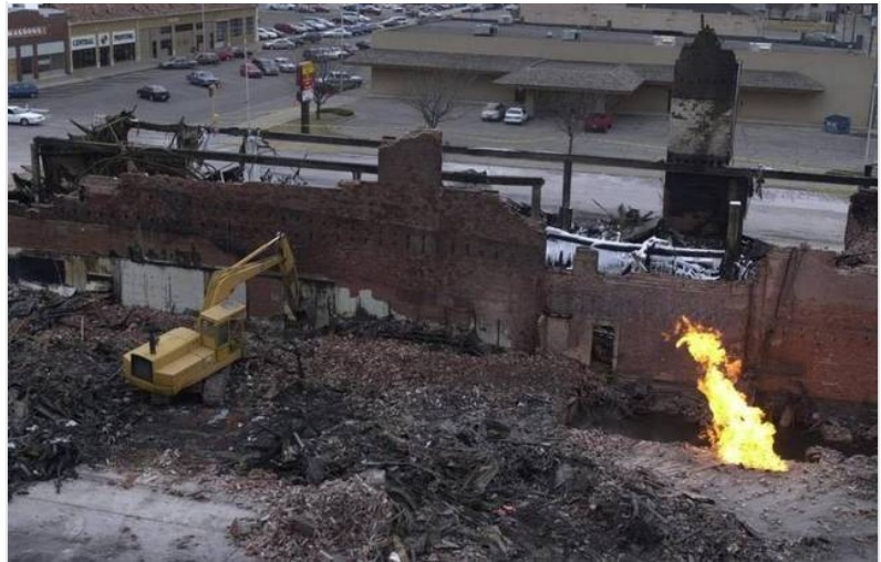
Figure 7. Photo of downtown Hutchinson, KS, after explosion from an underground storage field at Yaggy
