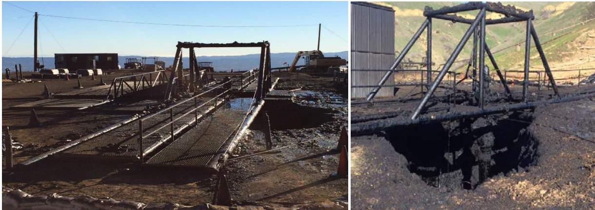
Figure 12. Vent crater caused by expulsion of top kill attempt materials
