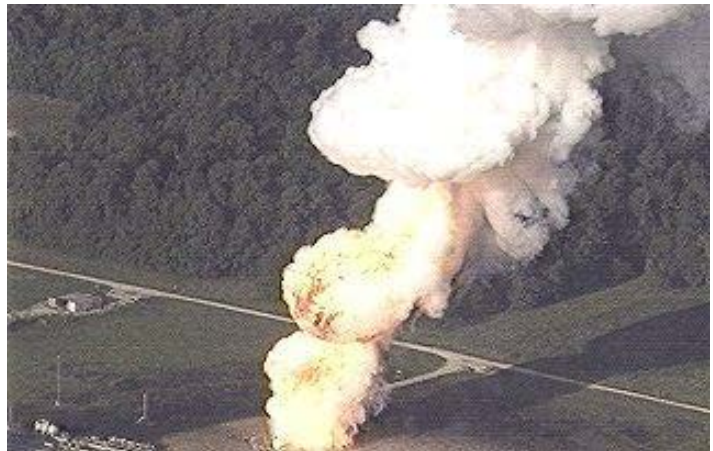
Figure 9. Uncontrolled gas release and fire at storage Cavern #1
