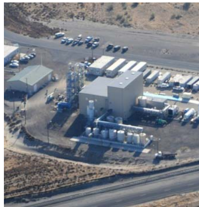
250K GPY IBR Facility Boardman, OR
