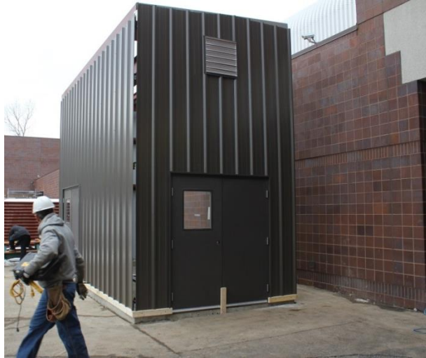
Biomass unloading building
