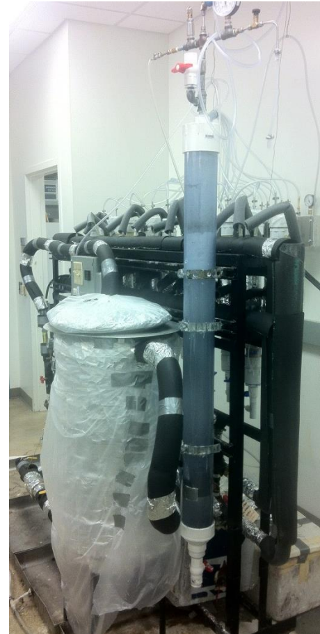
Cryovessel and CO 2 scrubber column
