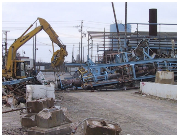
Figure 4.1.15-3: Photo of Standard Chlorine/Metachem Superfund Site, New Castle, DE (2006)
