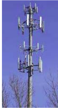
Figure 2.4.3-1: Monopole Cell Tower with Multiple Panel Antennas
